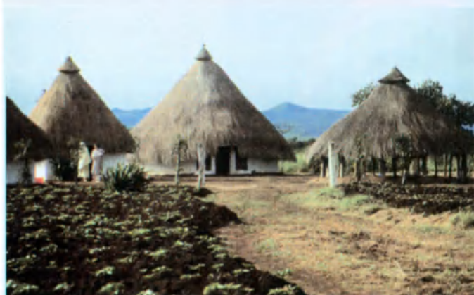
Dwellings constructed by Doudou, a well-known woman builder, in Ngaoundéré (Cameroon).
