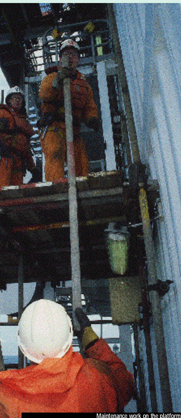
Maintenance work on the platform.
