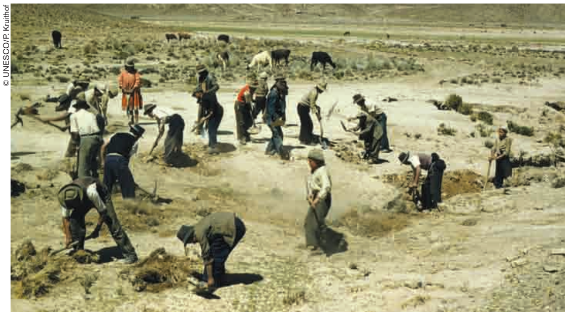
Building a road on the high plateaux of Bolivia.
