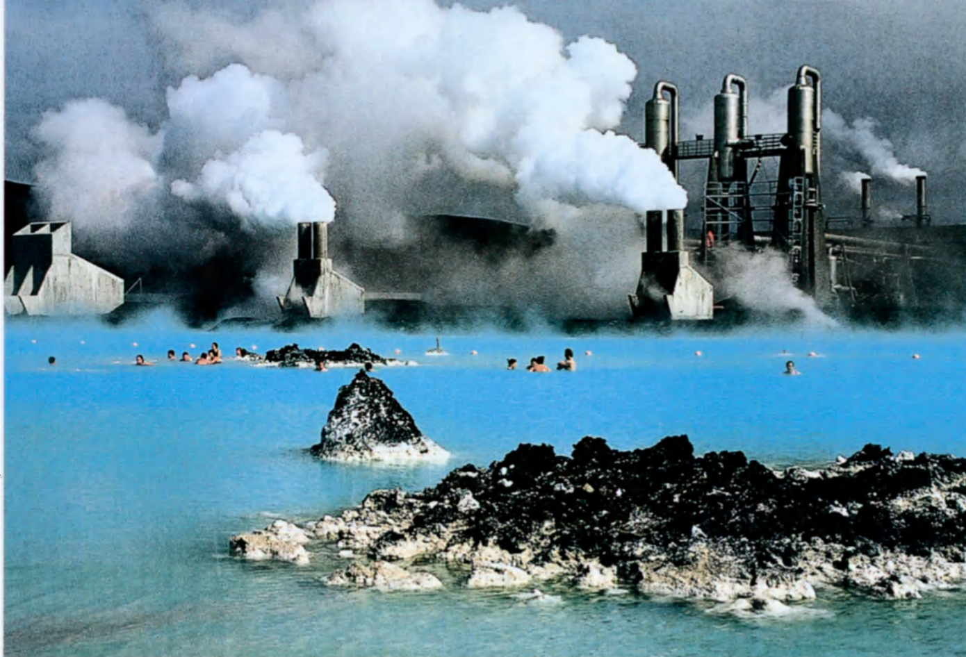
Svartsengi geothermal plant, above, provides Reykjavik with hot water. The diversion of its surplus production into a lava field has given rise to the Blue Lagoon (foreground), whose mineral-rich waters have a temperature varying from 25 to 35°C.
