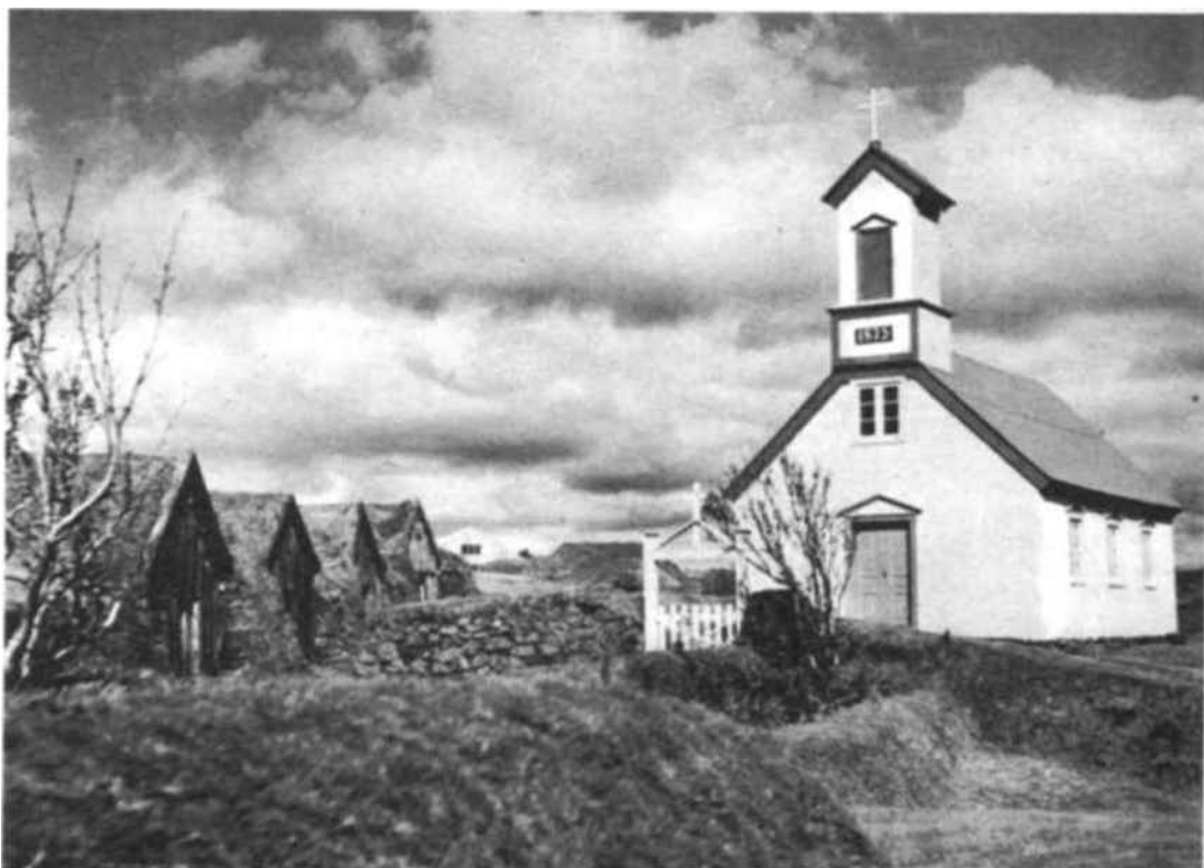
EVERY ROOM HAS ITS OWN ROOF The traditional Icelandic farm is built partly below ground level with a separate roof for each room. The row of roofs seen on the left of this photo all belong to one farmhouse and represent a link with old Viking architecture. Typical also is the form of the Lutheran church often found in Iceland's countryside. Newer houses are made of imported timber or concrete.
