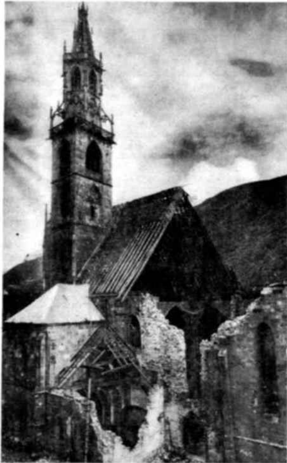
The competence with which partially war damaged buildings are being restored does great credit to Italian ingenuity. At Bolzano, for example, where the cathedral roof (above) suffered severe damage, the architects and experts charged with its reconstruction were faced with the problem of building material shortages, especially wood, when they began their work. As the photo (right) shows, they overcame this by replacing the ancient wooden beams with reinforced concrete.
