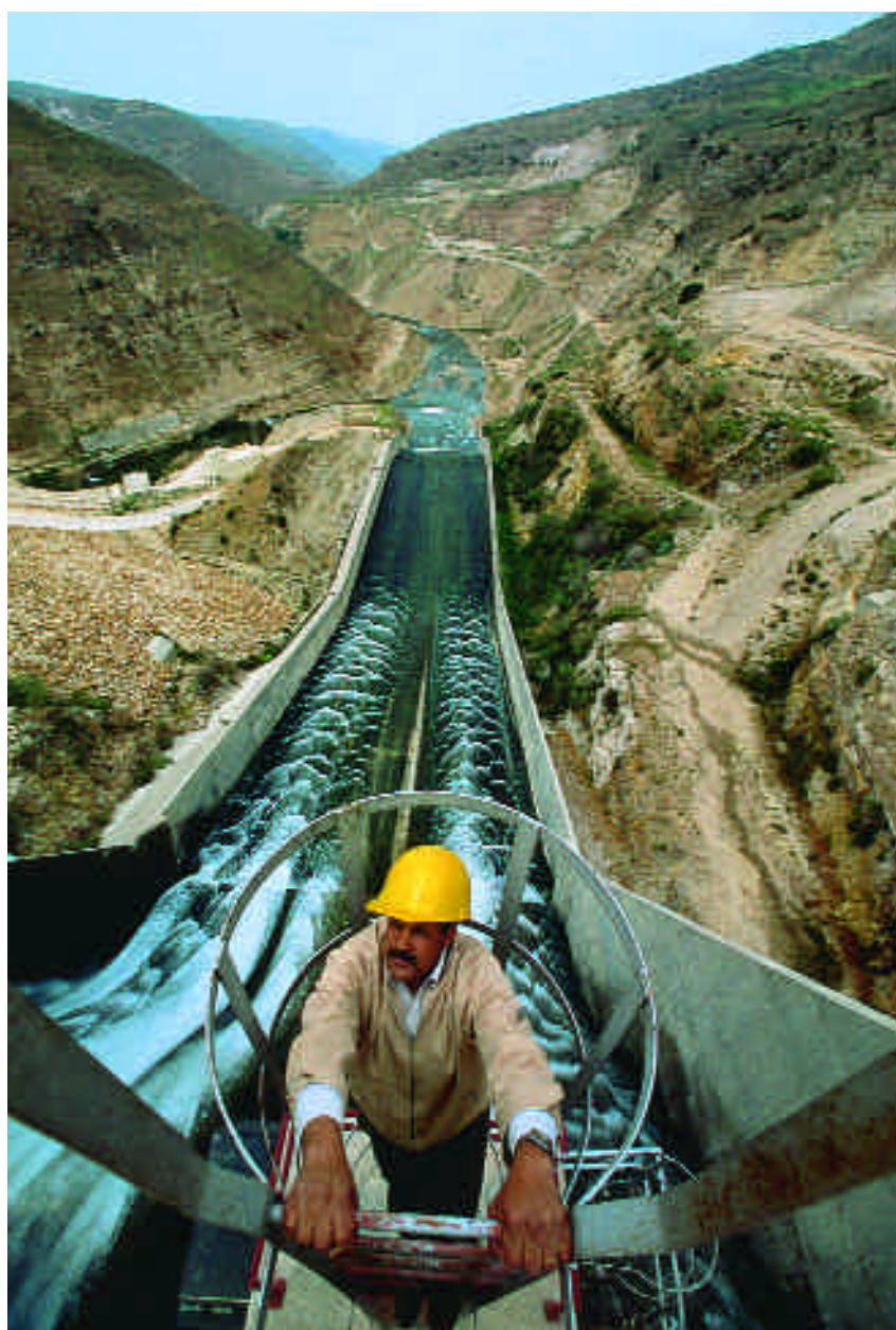
An engineer working on the King Talal dam, which supplies water to Jordan valley farms.
