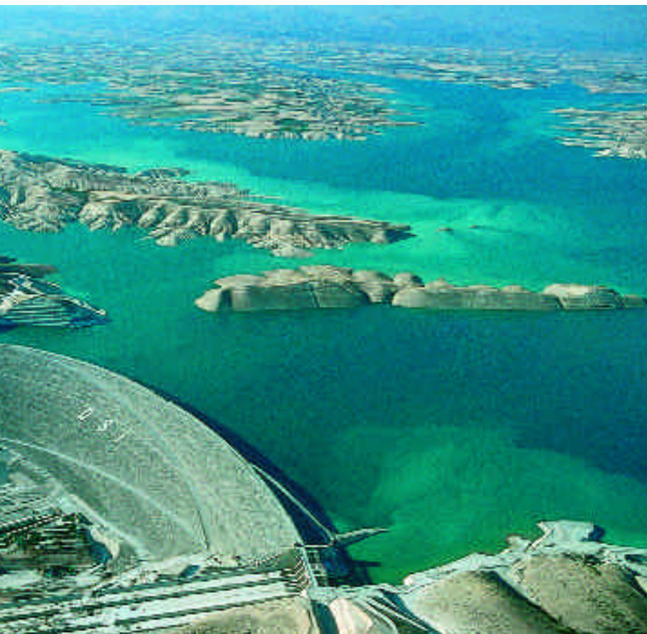
Aerial view of Turkey's Ataturk dam on the Euphrates.
