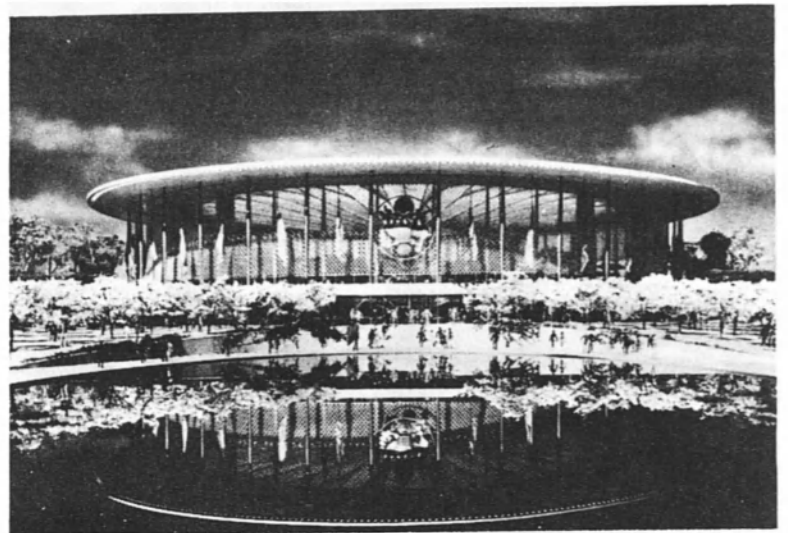
UNITED STATES PAVILION at Brussels Fair, 340 feet in diameter and 95 feet high, will be world's largest circular building without any interior columns. One of the remarkable features of this building is its "bicycle wheel" suspension roof of plastic attached to an inner metallic rim with high tension steel cables.
