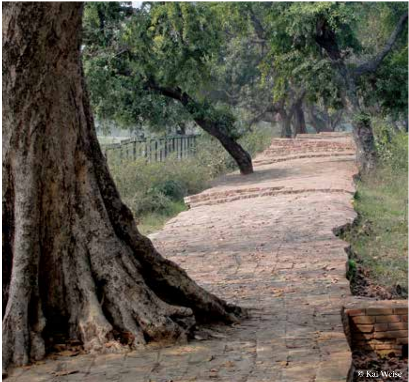
Fortification wall of Tilaurakot
