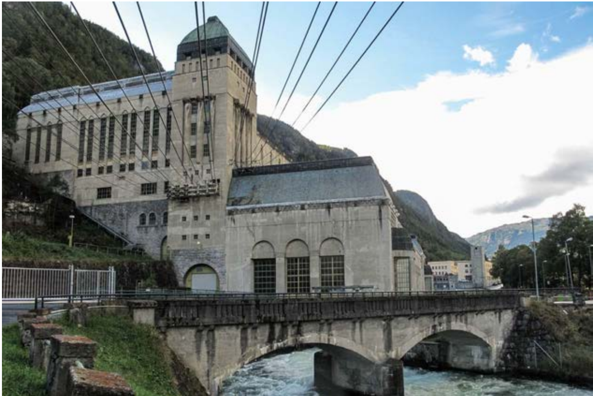
Såheim Power Plant
