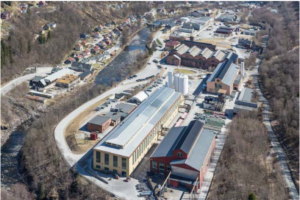
Rjukan, Hydro Industrial Park
