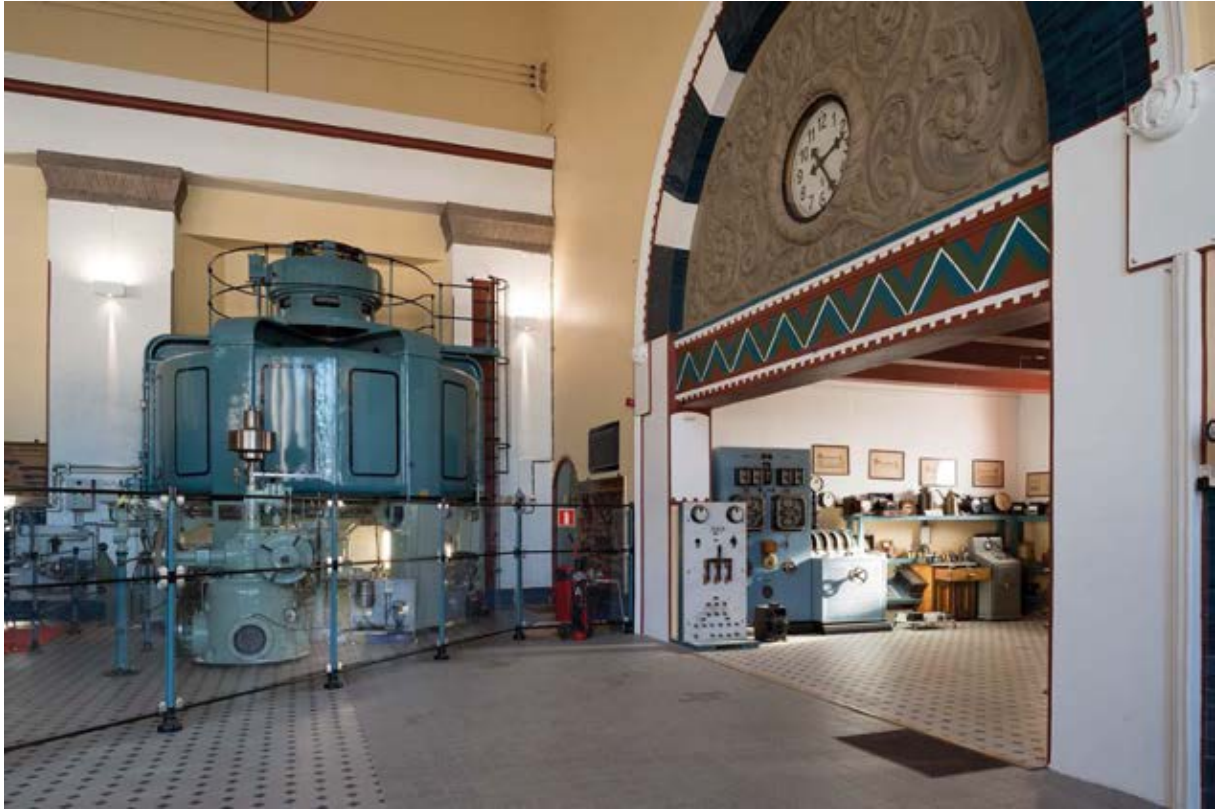
Tinfos II Power Plant
