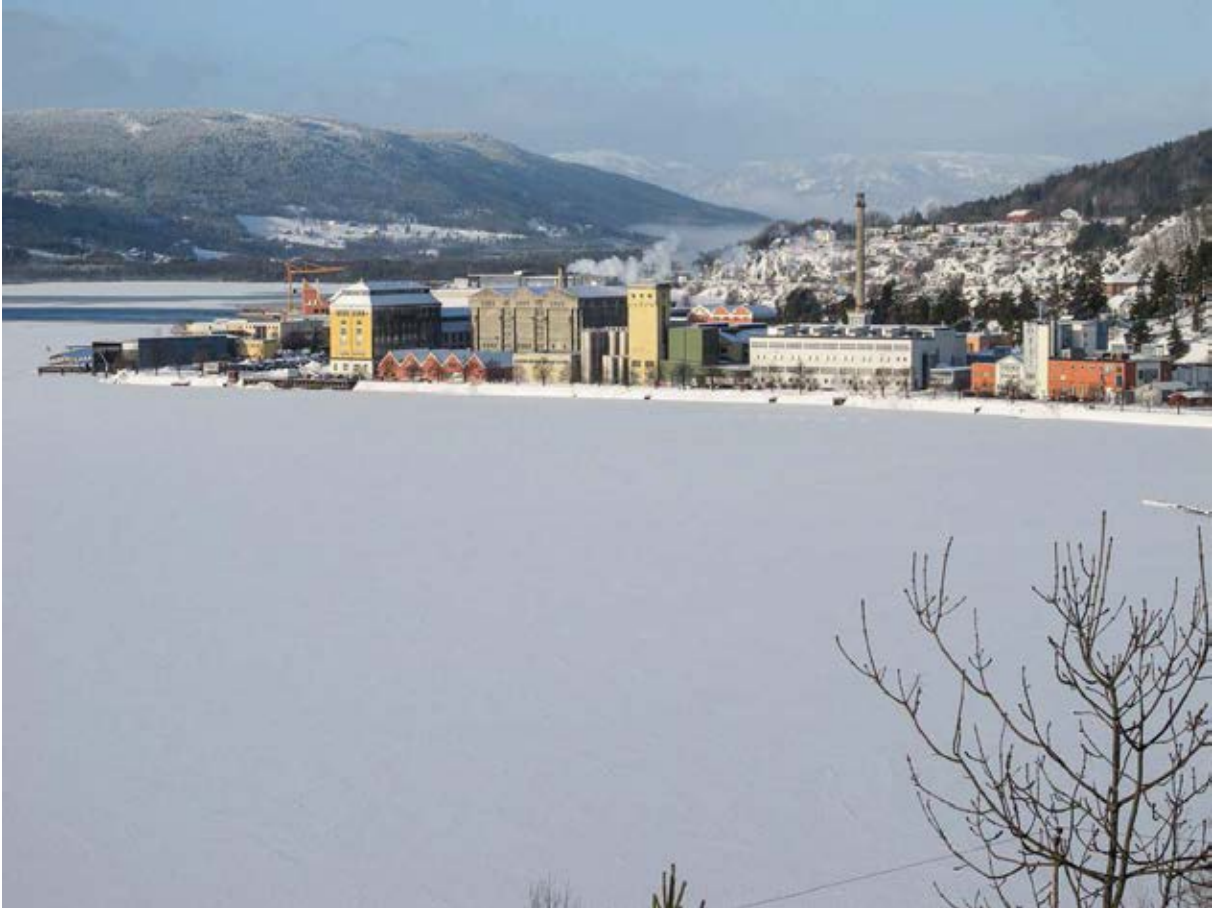
Notodden, Hydro Industrial Park
