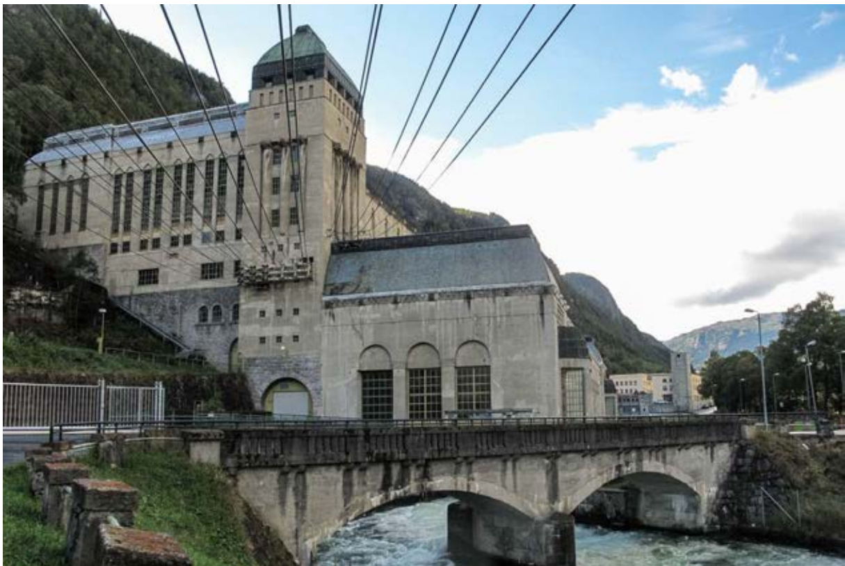
Såheim Power Plant
