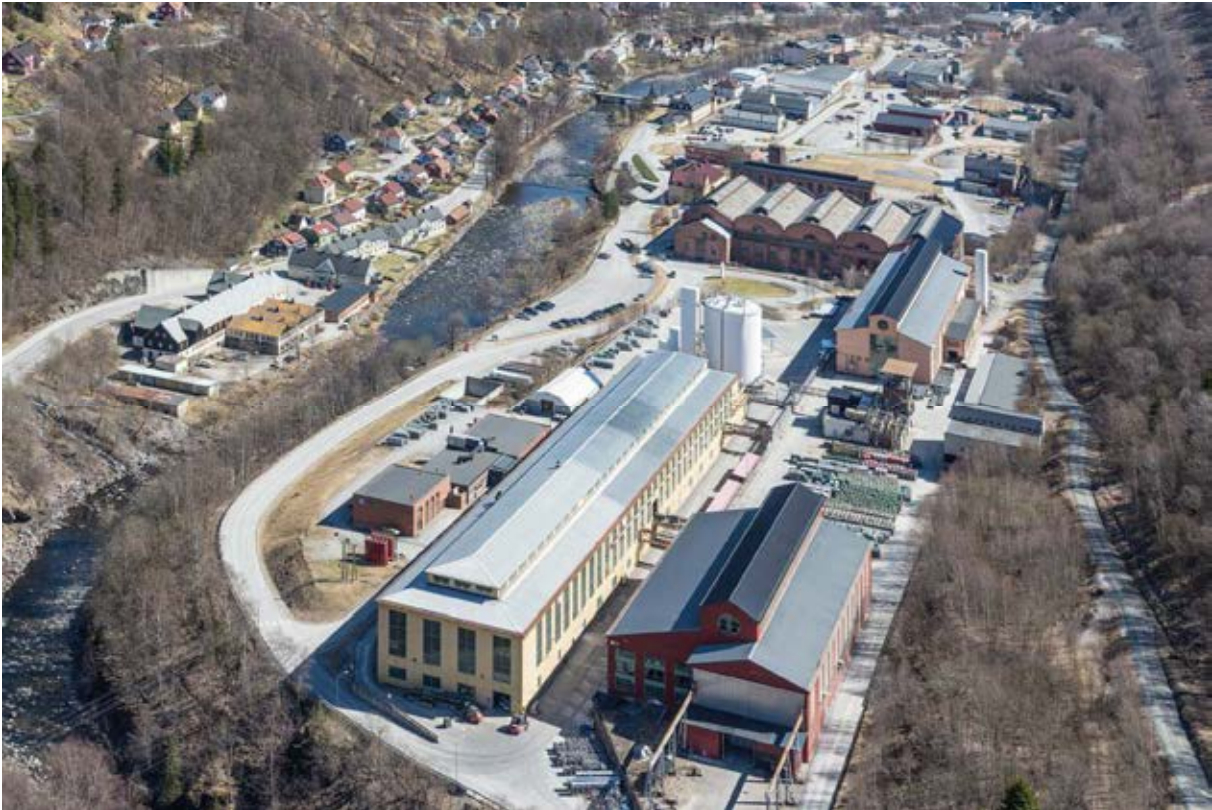
Rjukan, Hydro Industrial Park
