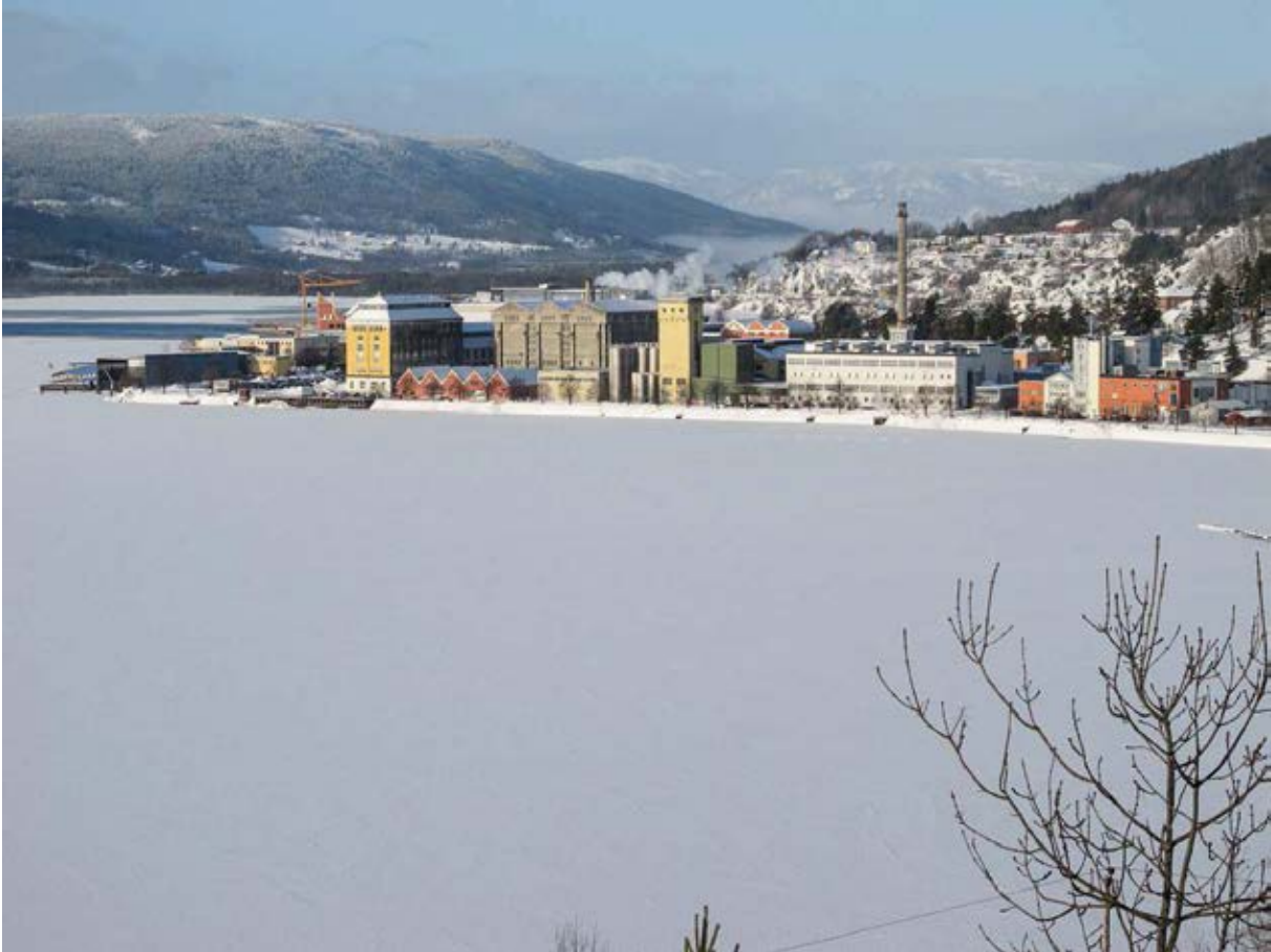
Notodden, Hydro Industrial Park
