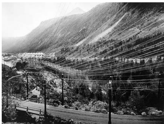
Power transmission from Vemork to the industry area in 1912. Photo: Anders B. Wilse.
