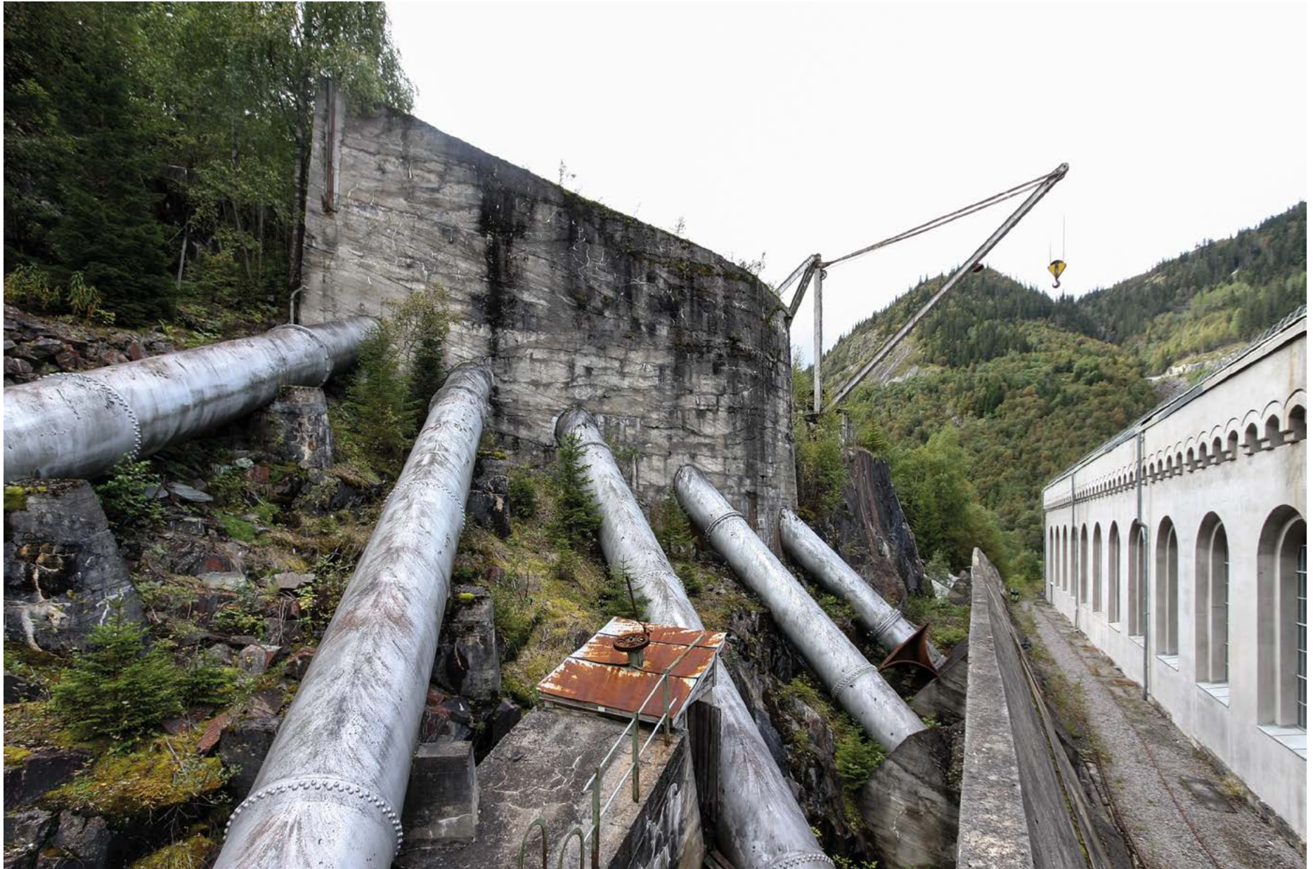
Fig. 22 Penstock and Vemork railway track at Vemork Power Plant. Photo: Eystein M. Andersen
