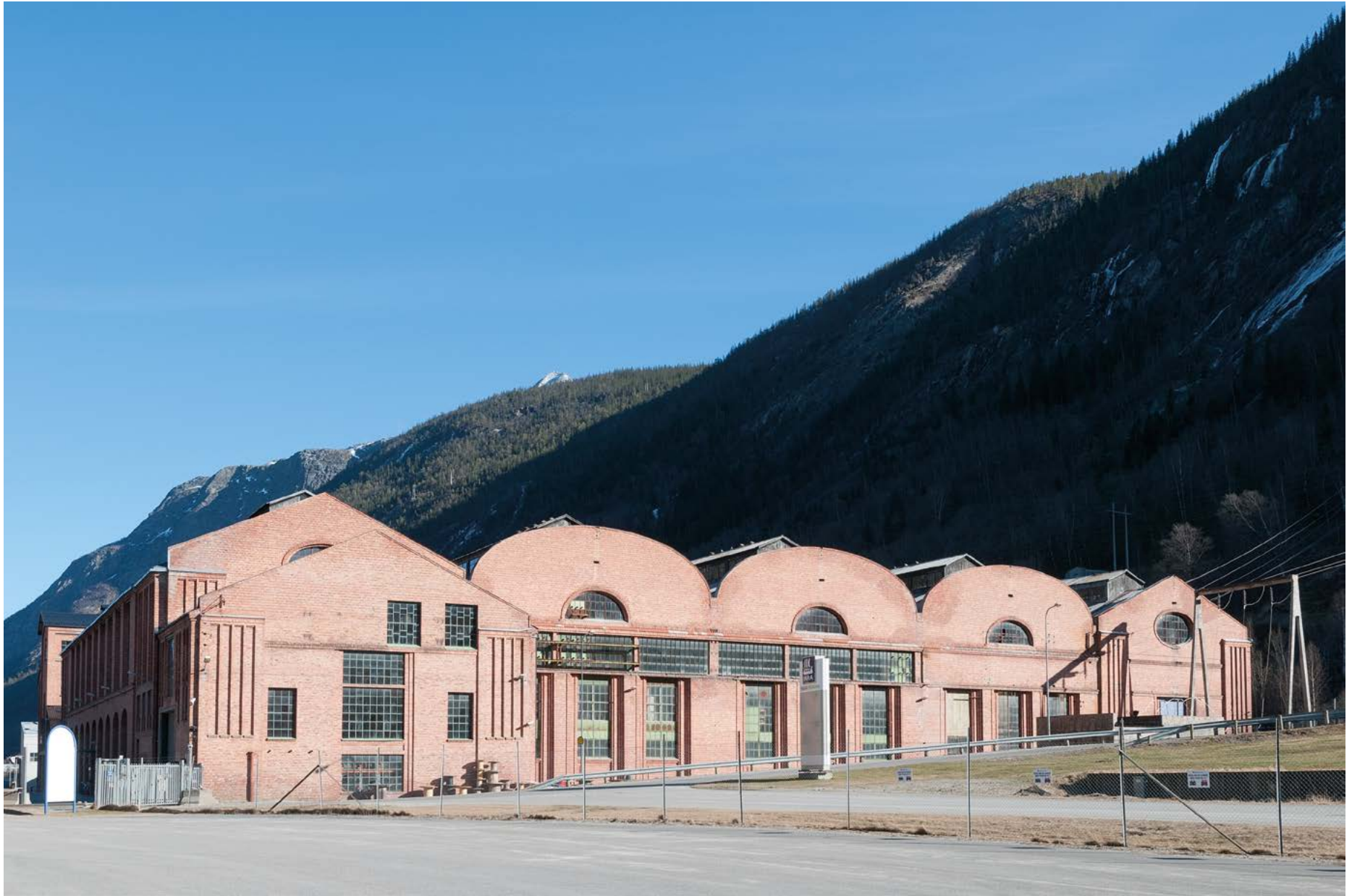
Fig. 58 Furnace House I, Hydro Industrial Park in Rjukan. Photo: Per Berntsen
