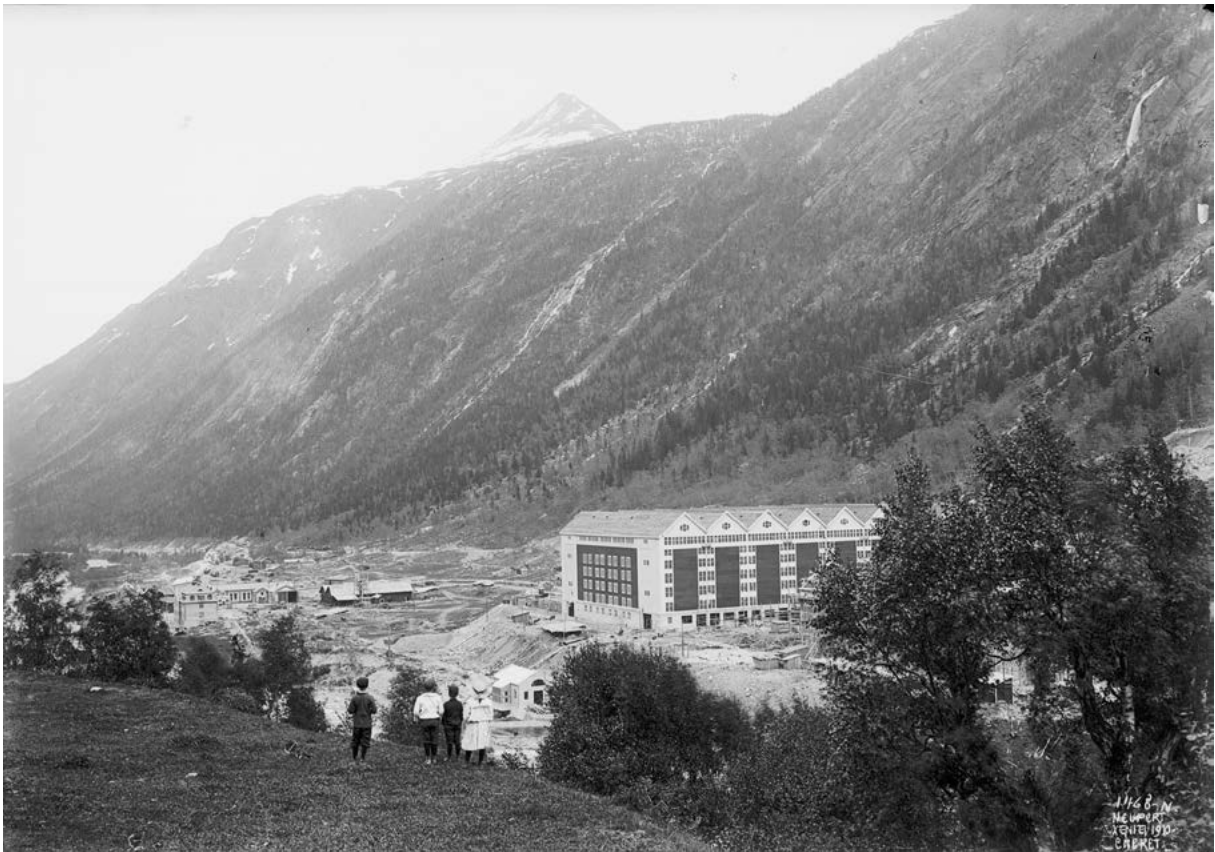
Tower house for the Rjukan I plant emerges on former grassland. Photo: Neupert.
