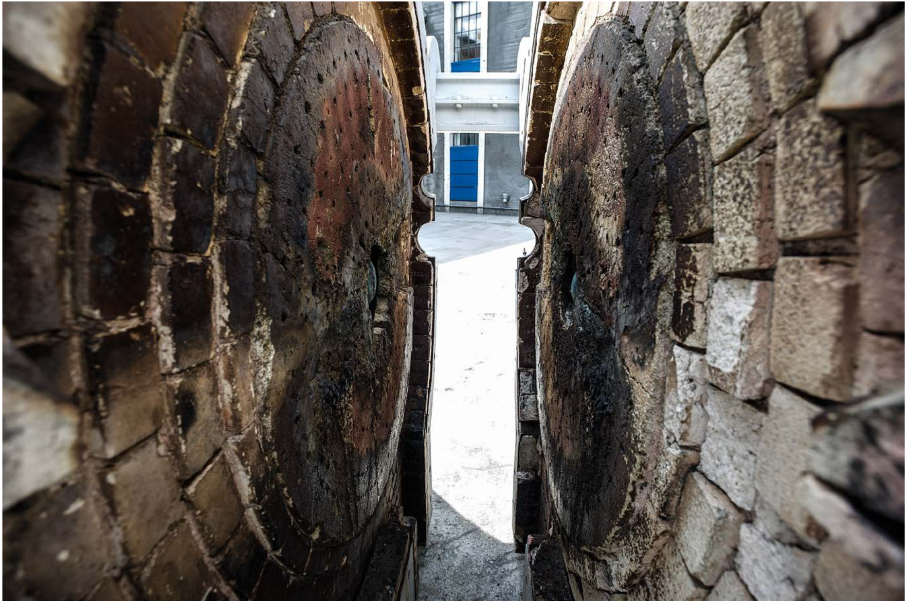
Fig. 52 Electric Arc Furnace, Notodden. Photo: Dag Jensen
