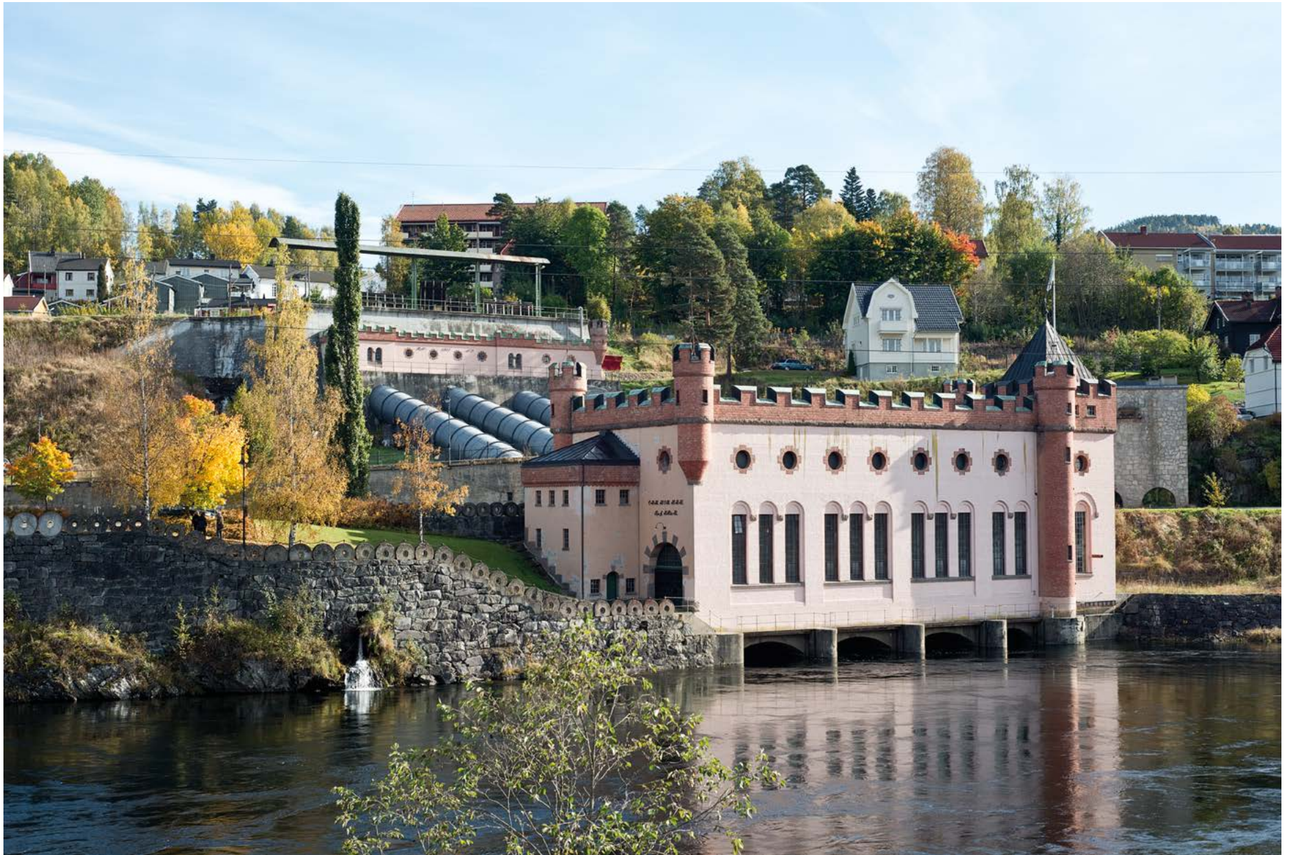
Fig. 12 Tinfos II Power Plant. Photo: Per Berntsen
