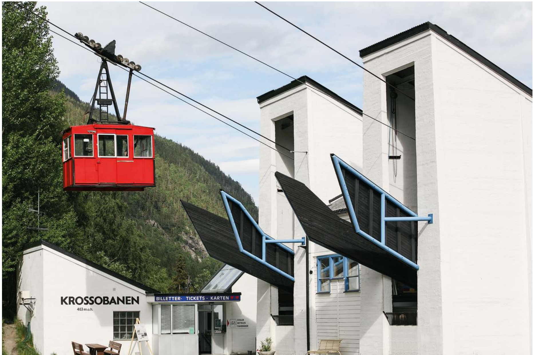
Fig. 93 Krosso Aerial Cableway, Rjukan Hydro Town. Photo: Hans Dieter Flegler
