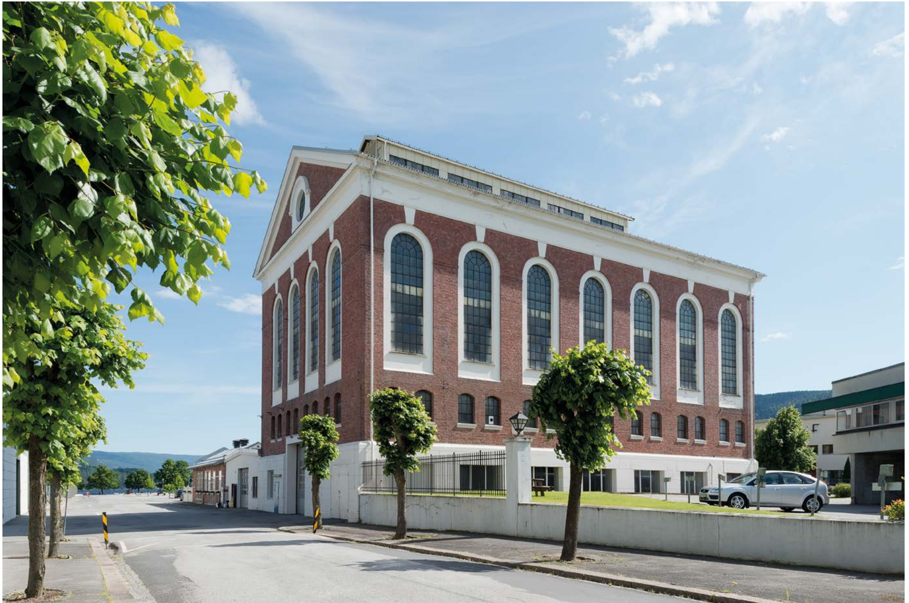
Fig. 46 Furnace House C, Hydro Industrial Park in Notodden. Photo: Per Berntsen
