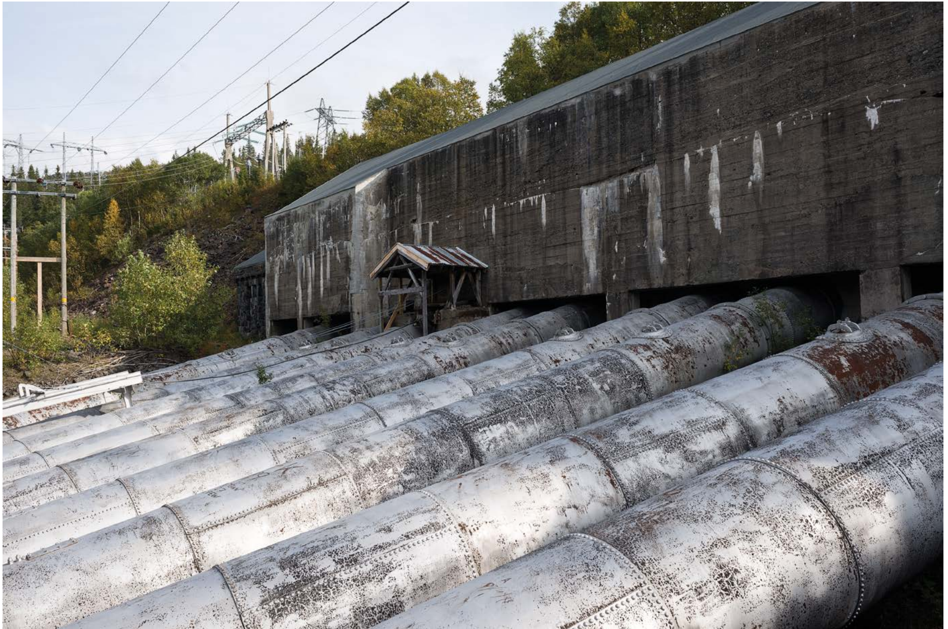
Fig. 20 Penstock valve house at Vemork Power Plant. Photo: Per Berntsen
