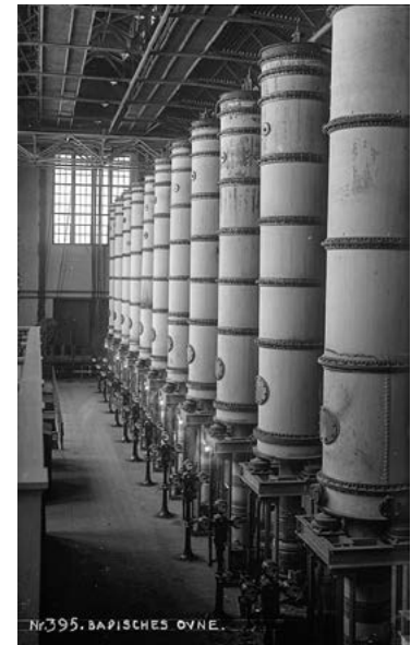
Furnace House I in 1910 to the left and part of its interior with Schönherr furnaces a few years later to the right. Photos: Norwegian Industrial Workers Museum.
