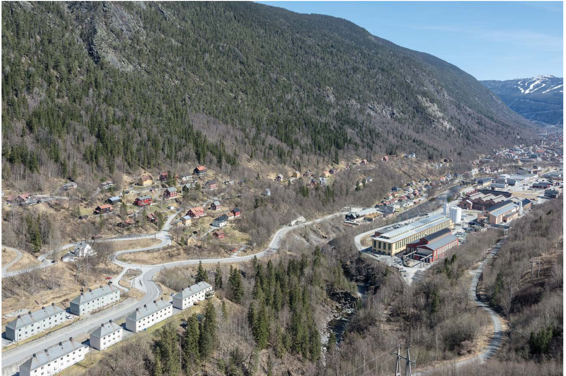
Fig. 94 Krosso and Villaveien-Flekkebyen housing areas, Rjukan Hydro Town. Photo: Per Berntsen
