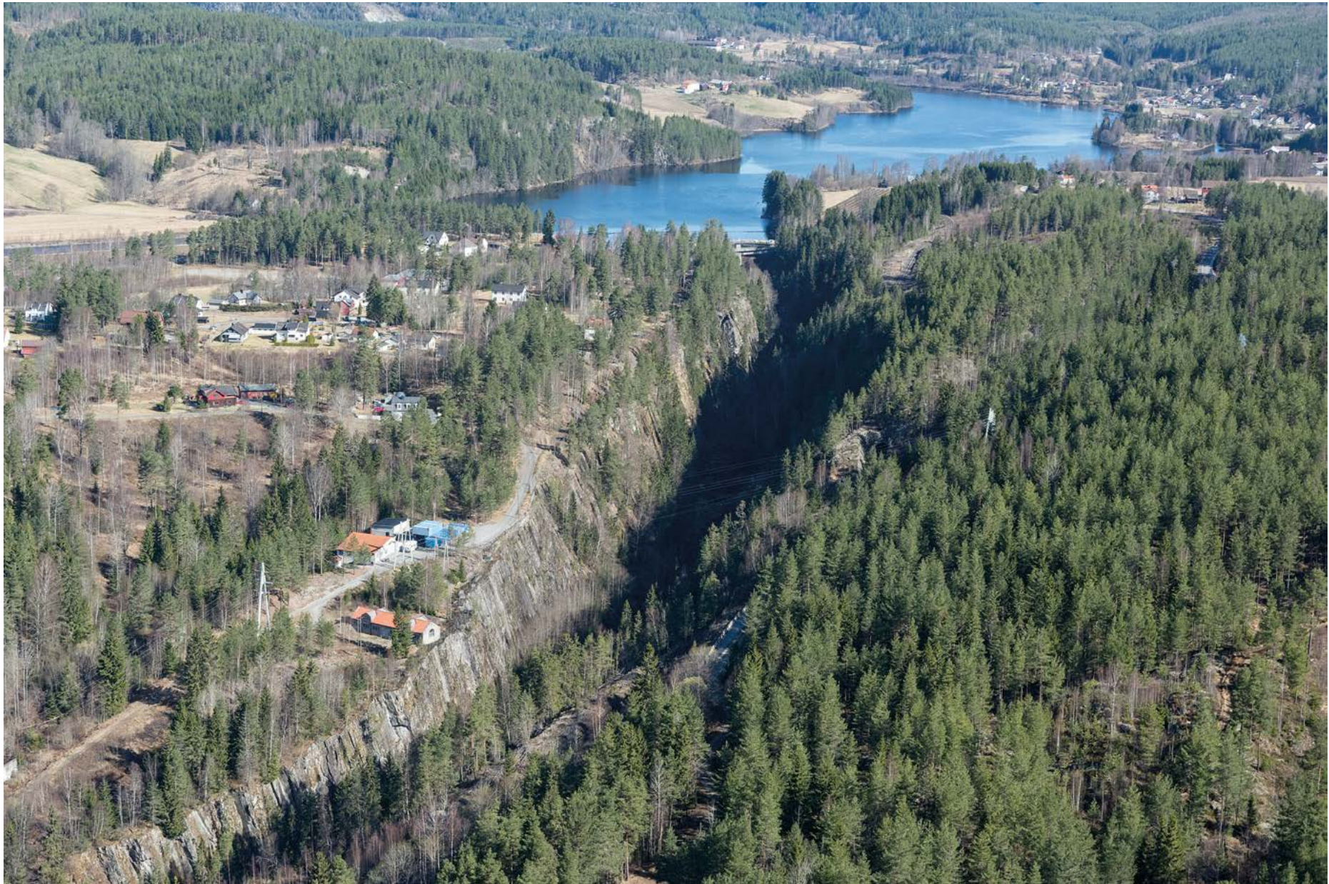
Fig. 15 Svelgfoss gorge with the Lightning Arrester House on the cliff. Photo: Per Berntsen
