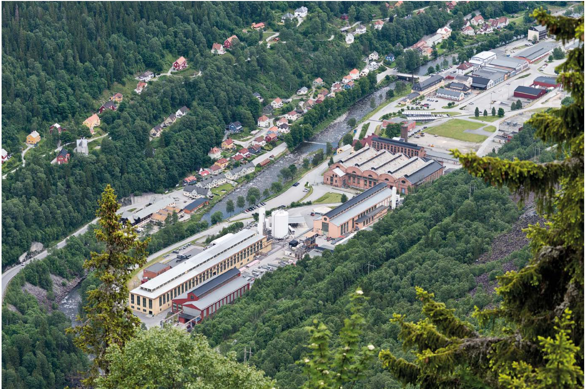
Fig. 54 Hydro Industrial Park in Rjukan. Photo: Per Berntsen
