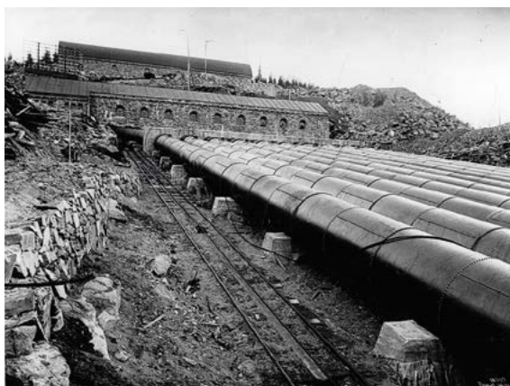
To the left: Penstock and valve house when finished 1912. Photo: Anders B. Wilse.
