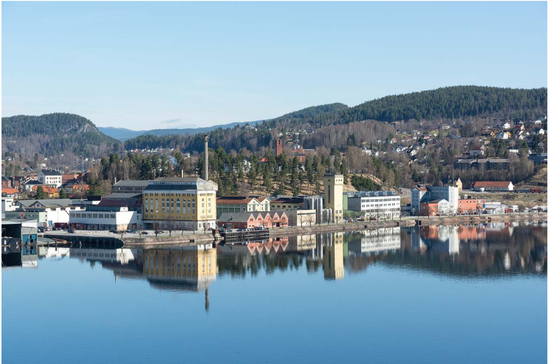
Fig. 40 Hydro Industrial Park in Notodden facing north east. Photo: Per Berntsen
