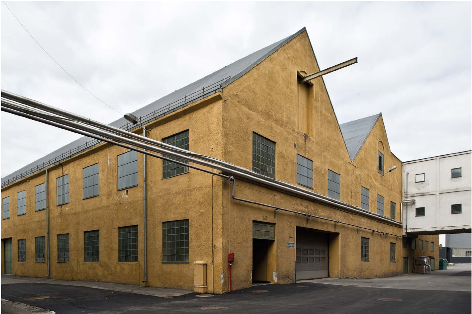
Fig. 47 Packaging Factory, Hydro Industrial Park in Notodden. Photo: Per Berntsen
