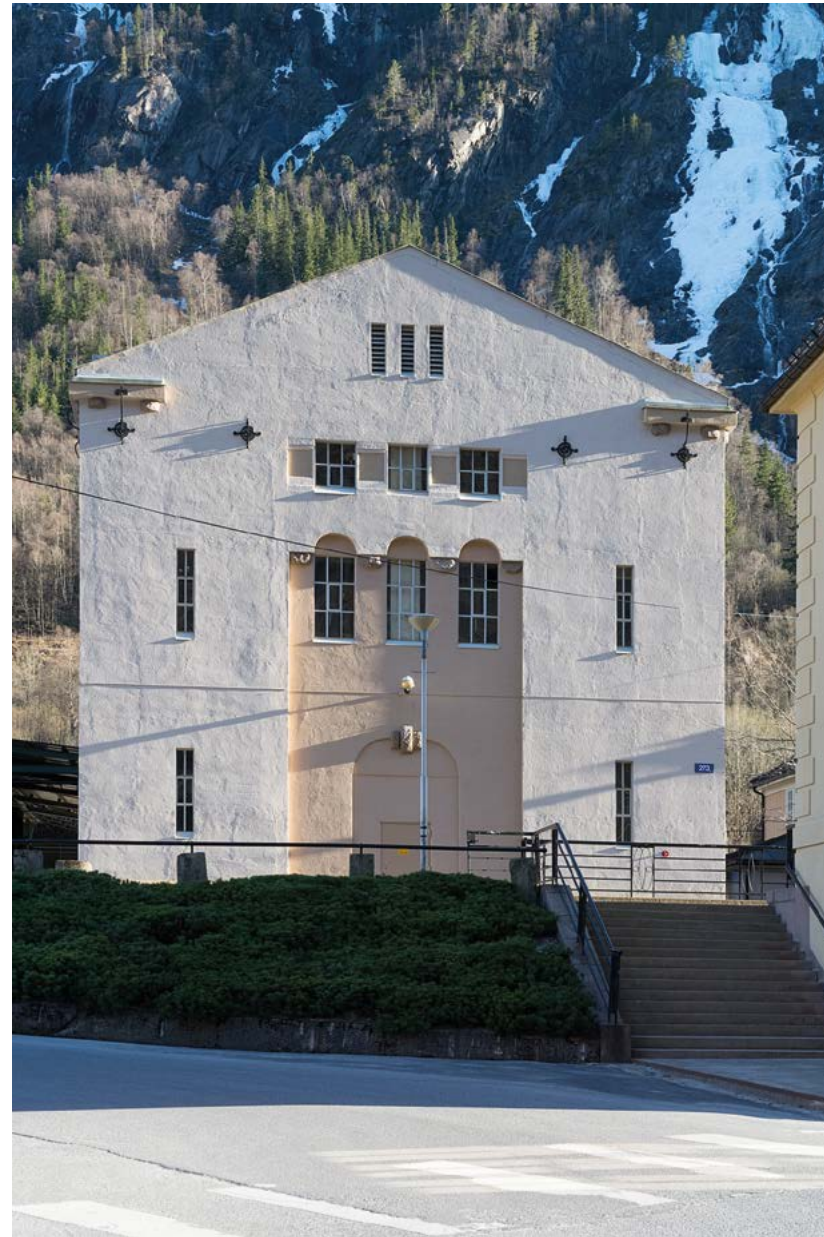
Fig. 38 Transformer and distribution station, Rjukan. Photo: Per Berntsen
