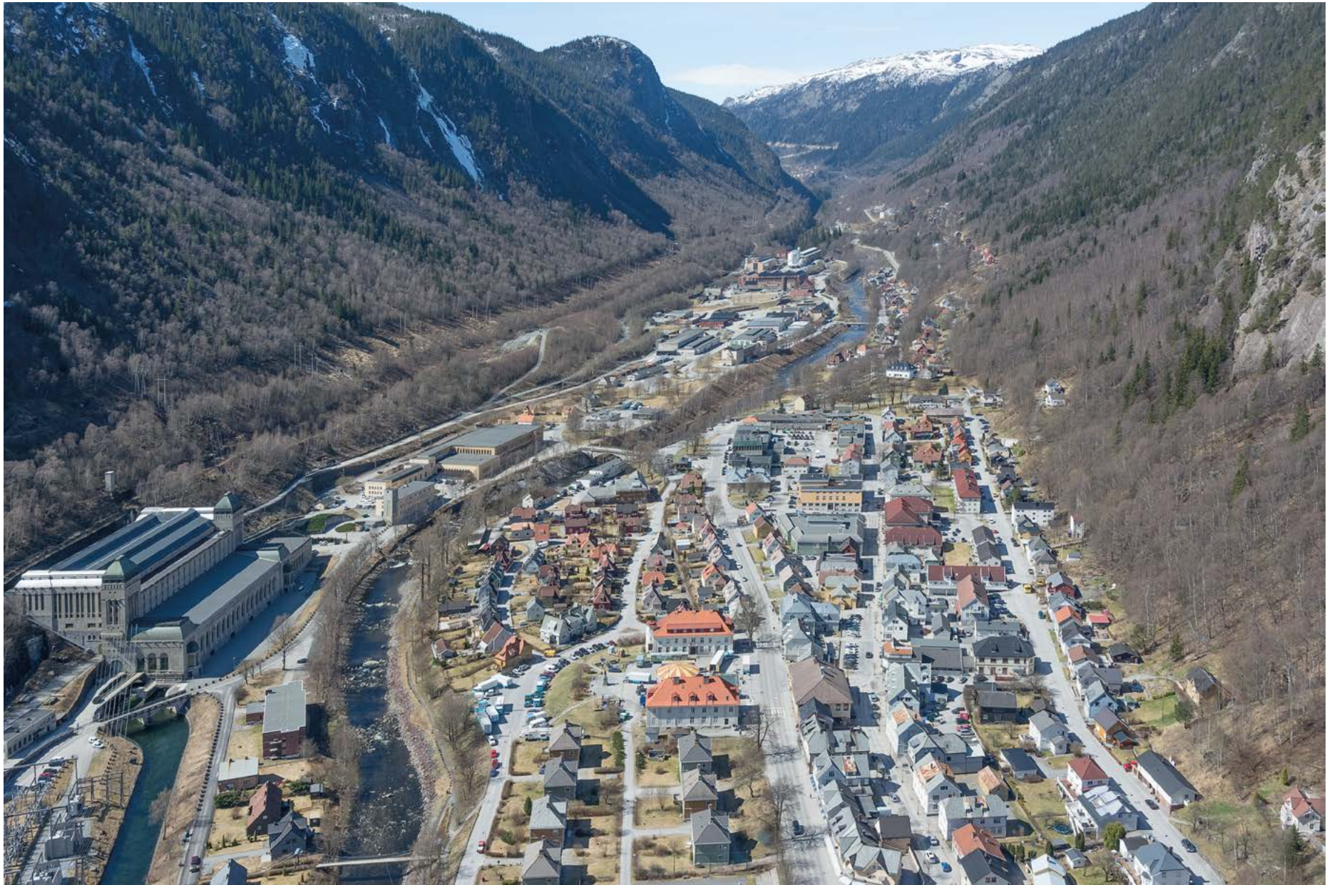
Fig. 110 New Town (house type O), Market Square and Tyskerbyen housing area facing west, Rjukan Hydro Town Photo: Per Berntsen
