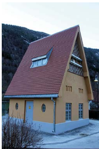
The Transformation station in Tyskerbyen has been restored back to its original appearance as seen in the top photo. Before and after the restoration below. Photo top: Anders Beer Wilse/ Norsk Folkemuseum Photo below left: Bjørn Iversen. Photo below right: Helge Songe.
