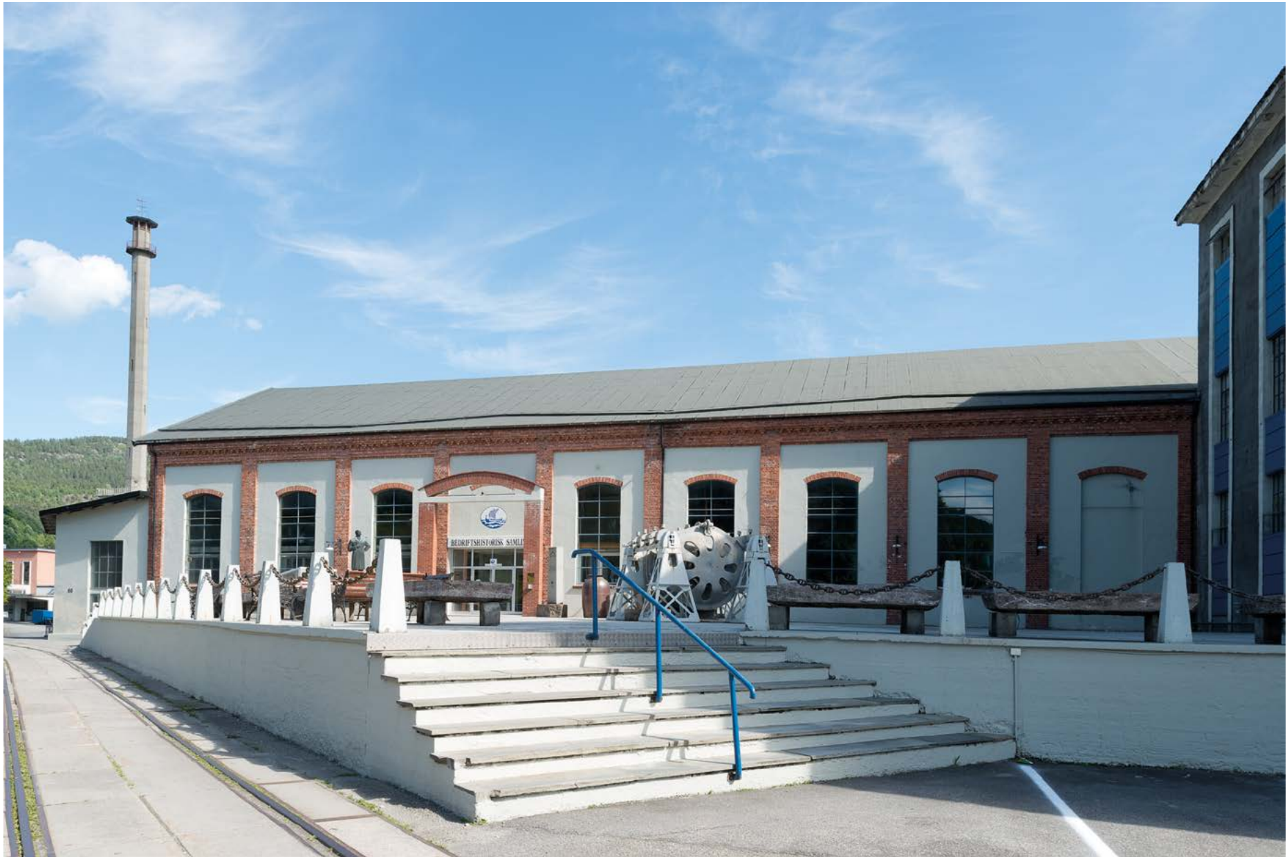
Fig. 43 Furnace House A, Hydro Industrial Park in Notodden. Photo: Per Berntsen
