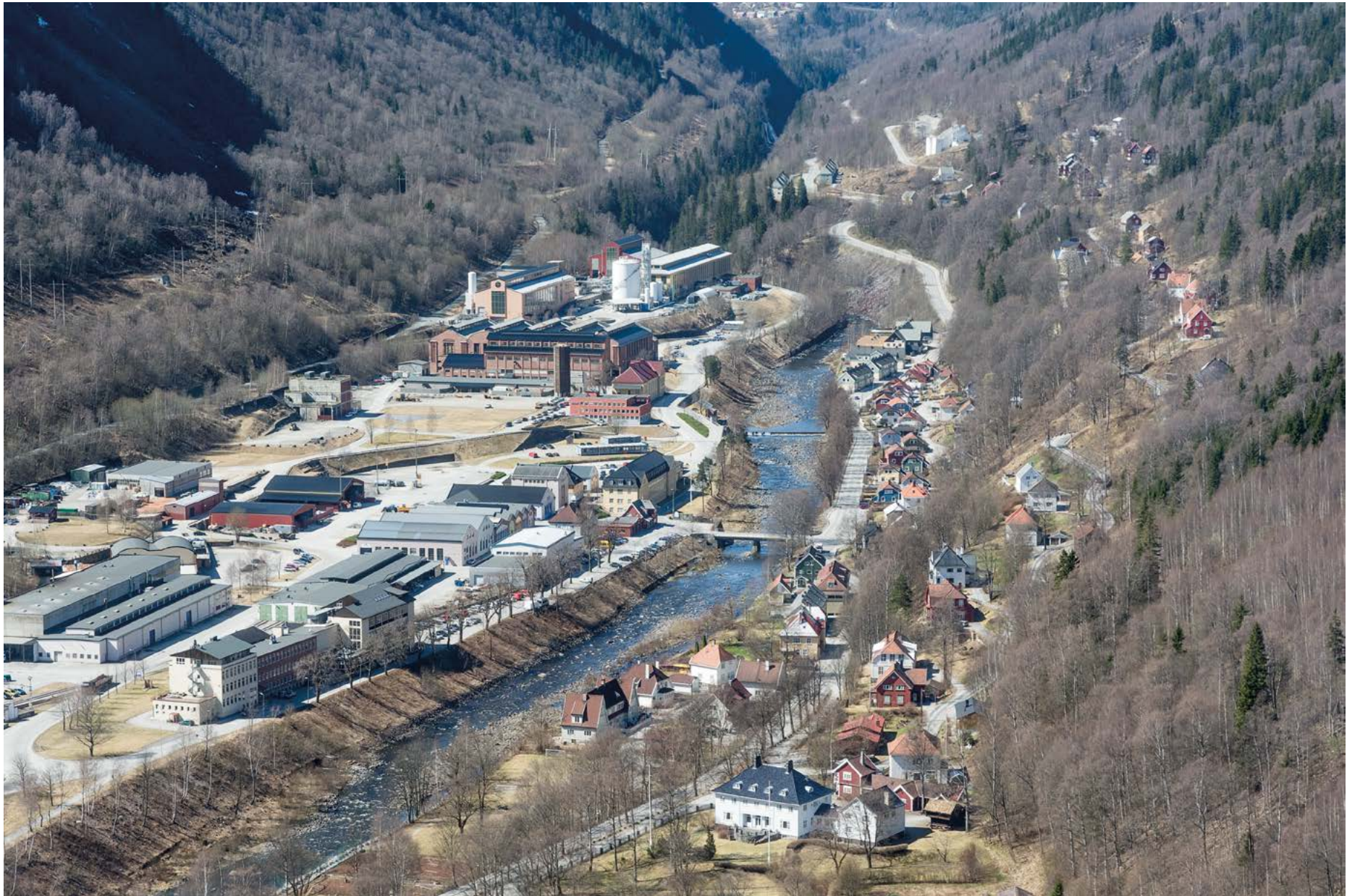
Fig. 97 Villaveien-Flekkebyen housing area with the industry area on the south bank, Rjukan Hydro Town. Photo: Per Berntsen
