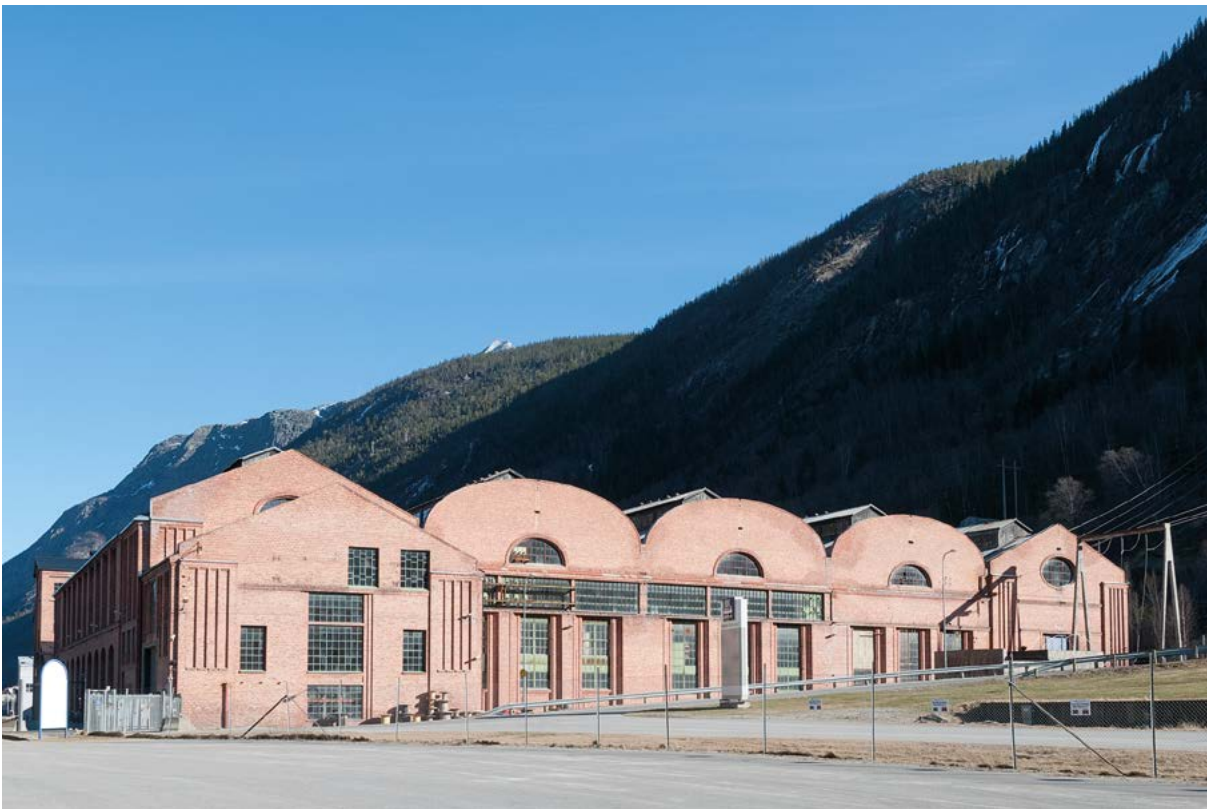
Furnace House I, west facade, today. Photo: Per Berntsen.
