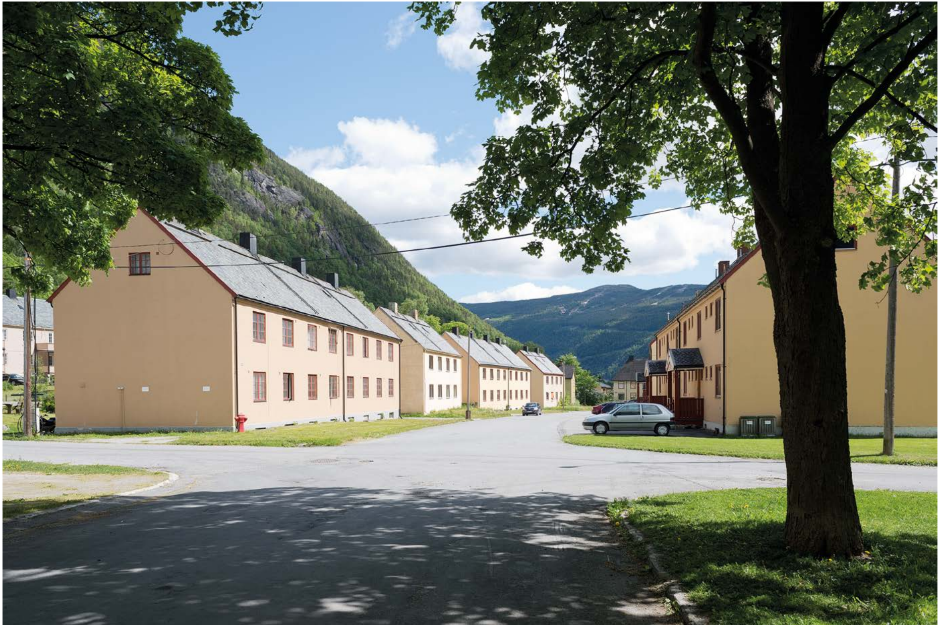
Fig. 116 Tveito Avenue, Rjukan Hydro Town. Photo: Per Berntsen
