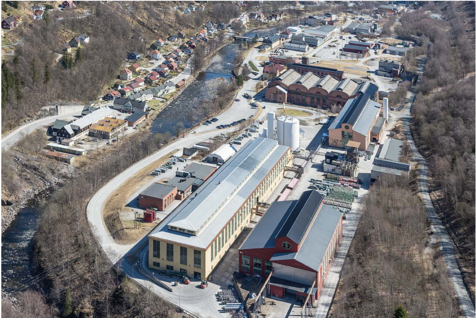
Fig. 55 Hydro Industrial Park in Rjukan. Photo: Per Berntsen
