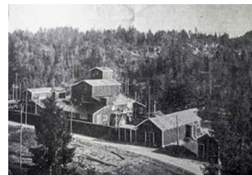
Vassmoen near Arendal, birth-place of Sam Eyde and where he was involved in the harnessing of waterfalls in Nidelva river.
