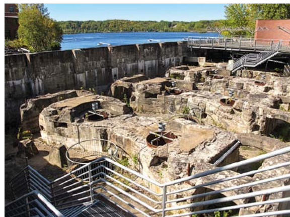
In Shawinigan the ruin of Alcan 16 power plant that was demolished in 1946 shows concrete structures for leading the water to and through the turbines, as part of the theme park. Photo: Trond Taugbøl.
