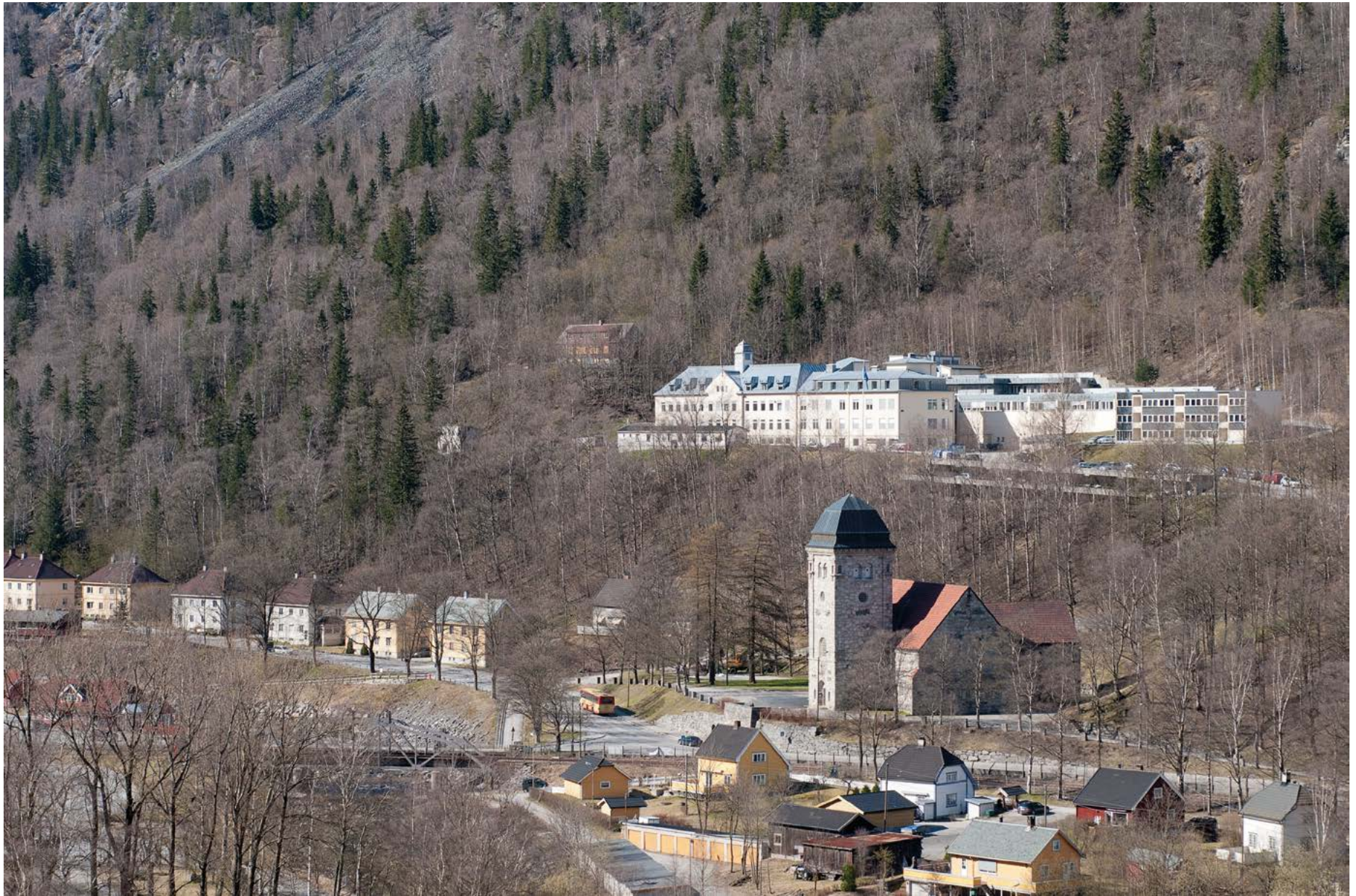
Fig. 108 Rjukan Church and Rjukan Hospital, Rjukan Hydro Town. Photo: Per Berntsen
