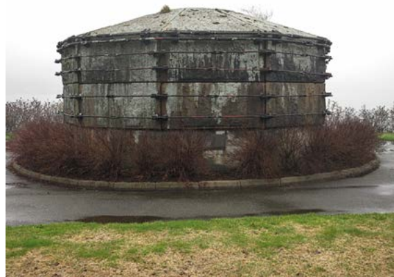
The top of one absorption tower is placed as a memory of the altogether 71 that were in place at Herøya between 1929 and 1982. Their height was 30 meters, weighing 26.000 tons and containing 13.000 granite blocks. Photo: Trond Taugbøl.
