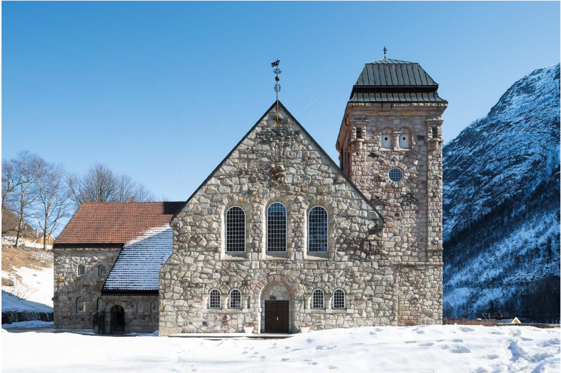
Fig. 109 Rjukan Church, Rjukan Hydro Town. Photo: Per Berntsen
