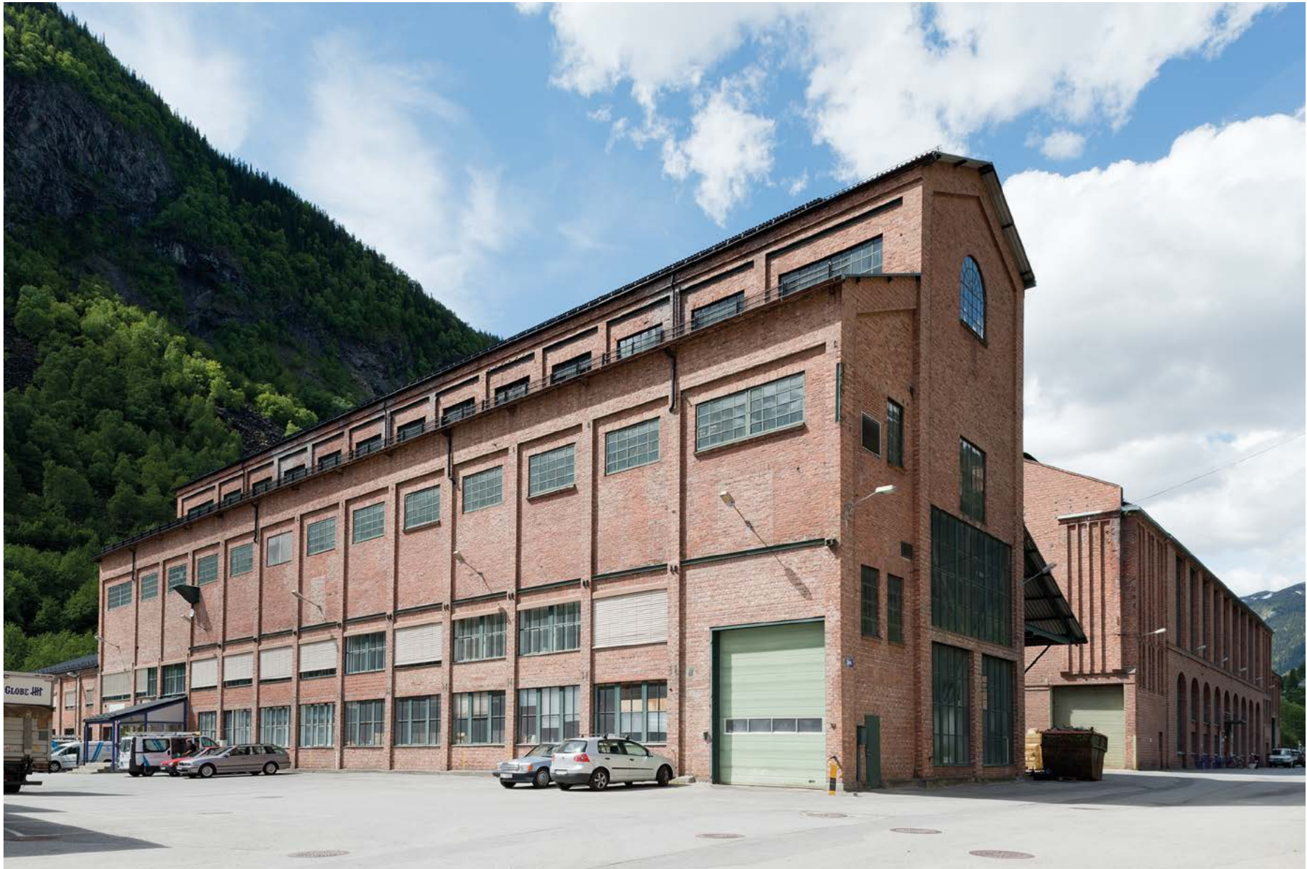
Fig. 59 Boiler House, Hydro Industrial Park in Rjukan. Photo: Per Berntsen
