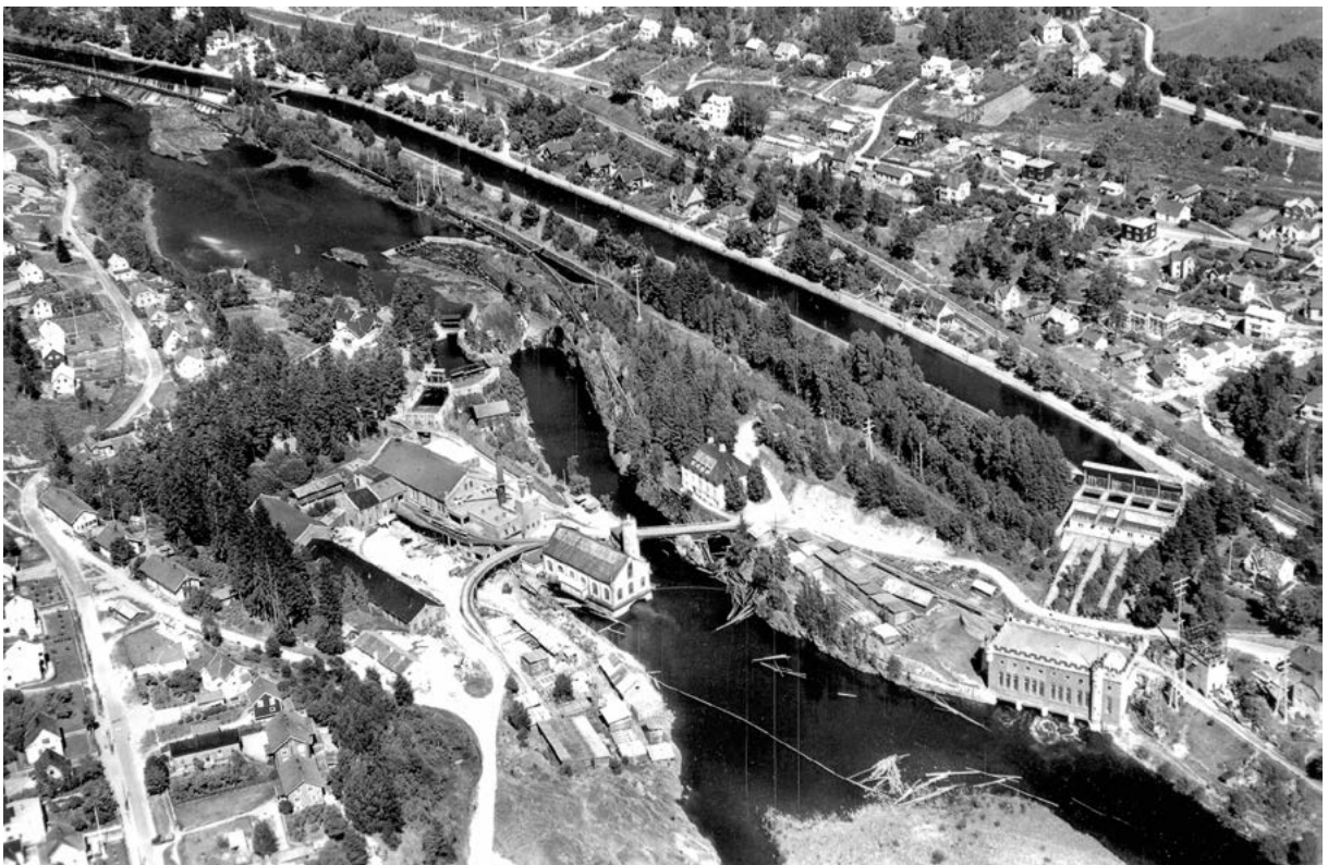
The area with Tinfos I and II with the Holta Canal seen from the air before 1955. Photo: Notodden Municipality.
