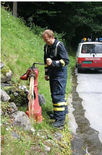
To the left: Some fire hydrants of the distinctive Rjukan type have been equipped with modern internal component as a trial project to preserve the hydrants instead of replacing them with new models.
