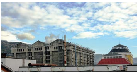
Tower House A under restauration in 2012. Photo: Eystein M. Andersen.
