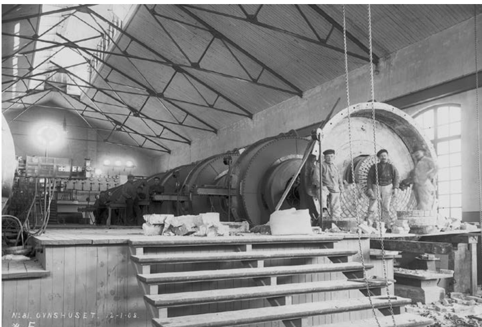
Interior of Furnace House A in 1908. New electric arc furnaces under construction. Photo: Norsk Hydro.
