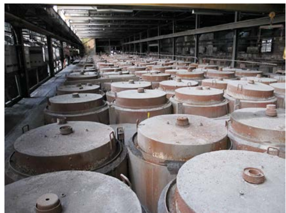
The more than 300 ovens of the Frank-Caro type in the Cyanamide factory are a unique feature at the Odda Smelteverk. Photo: Trond Taugbøl.
