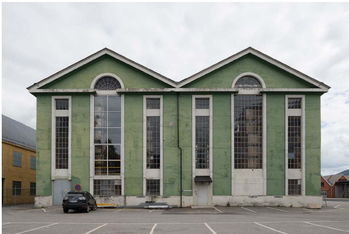
Nitrogen Plant and Gas Cleaning Plant. Photo: Per Berntsen.
