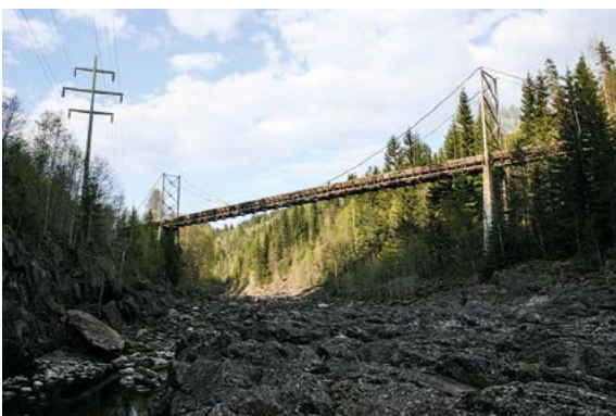
The timber flume crossing over Tinnelva river. Photo: Telemark County Council.
