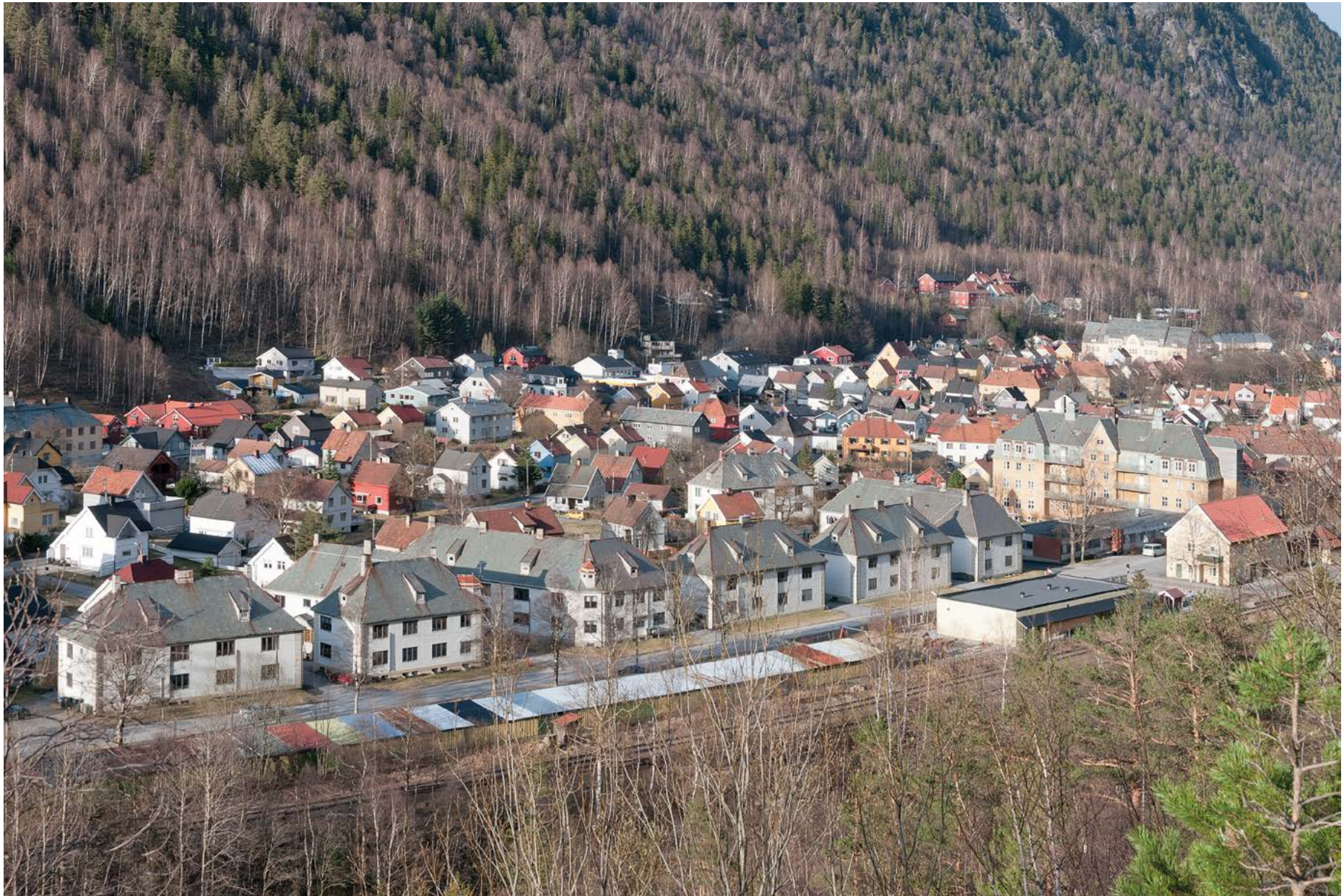
Fig. 111 Mannheimen single men's home and Paradiset housing complex, Rjukan Hydro Town. Photo: Per Berntsen
