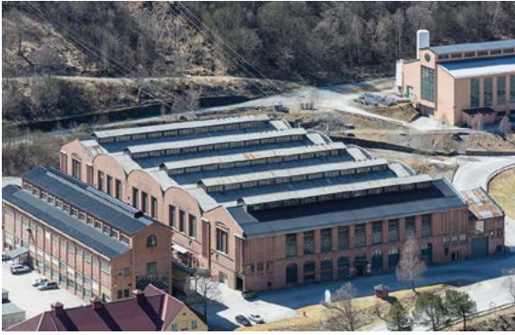
Furnace House I today. Photo: Per Berntsen.
