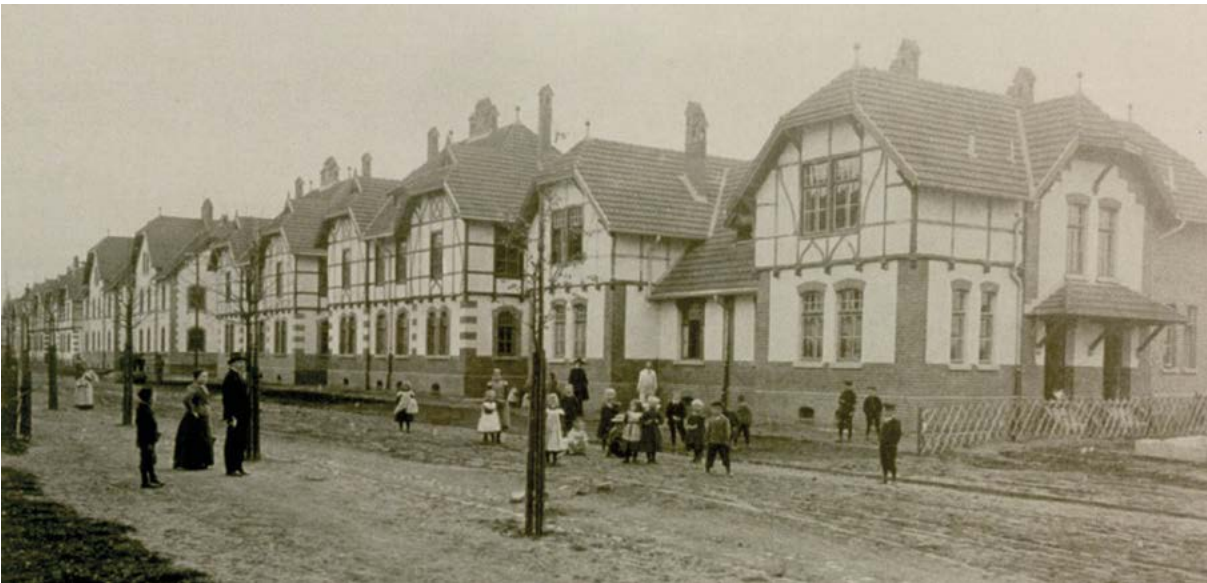
Workers homes on Vitalistrasse, Braunfeld, Germany, built 1902-03 by the gasworks on Widdersdorfer Strasse. Photo: www.Braunsfeld.info .
