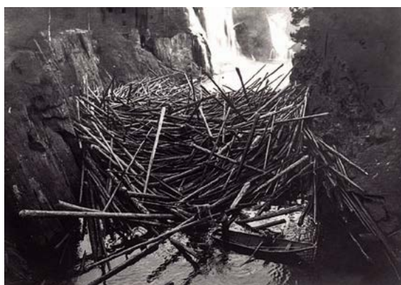
Timber floating. Trouble beneath Tinnfossen waterfall. Photo: Notodden Historielag.
