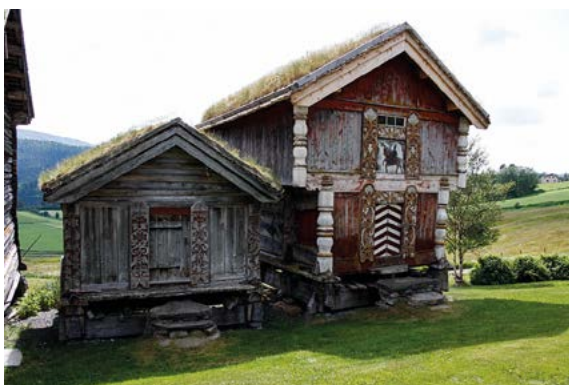
Traditional Telemark architecture, loft & bur (storage buildings) at the farm Mo Øvre in Vinje. Photo: Unn Yilmaz © Riksantikvaren.
