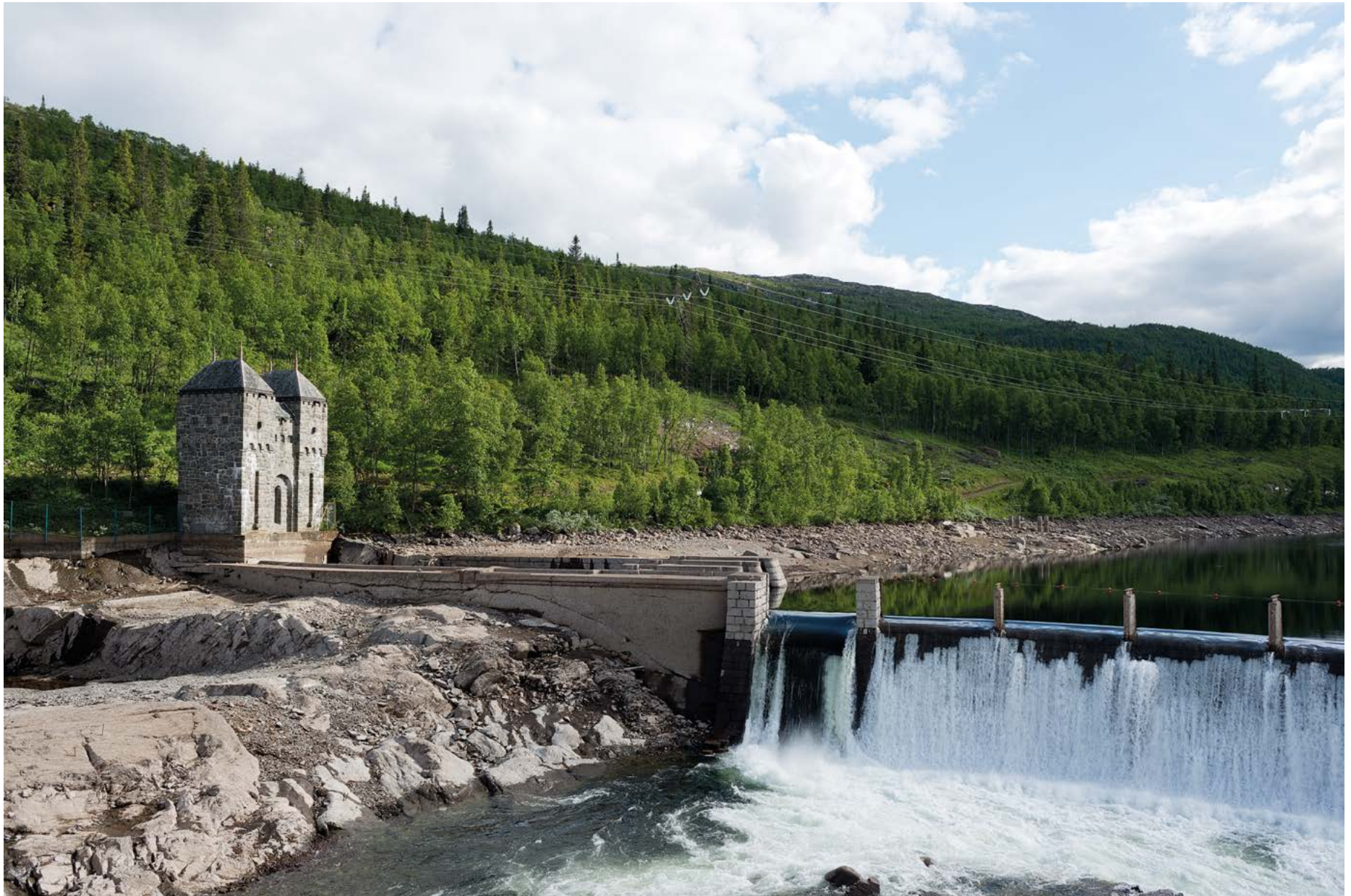
Fig. 18 Skarsfos Dam I with intake gate house. Photo: Per Berntsen
