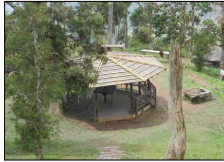
Gazebo repairs underway at Holywell
