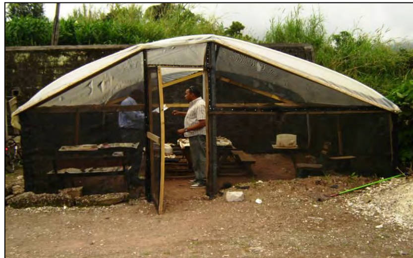
Cascade Community Greenhouse built under another project still in use by Cascade School
