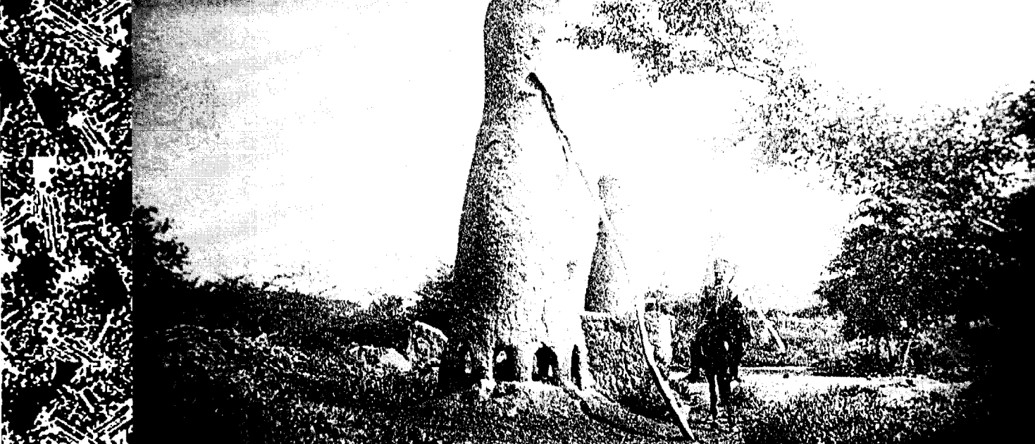
Metallurgy ovens of the Yatenga (relative scale from soldier on horseback).
