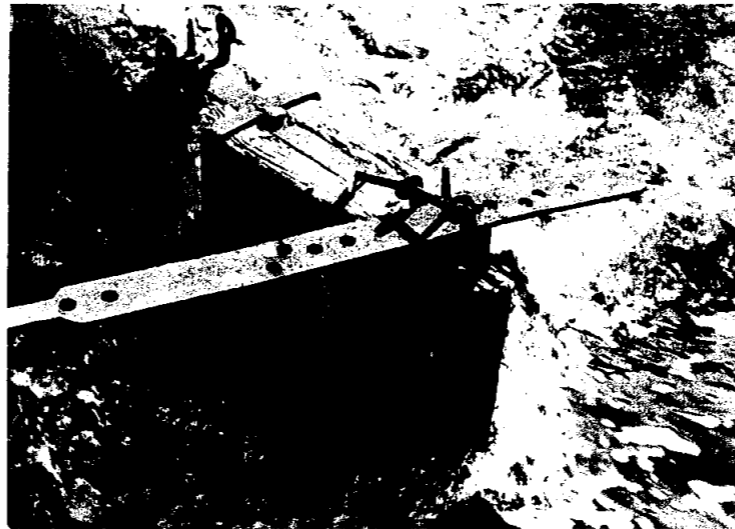
Mobile partidores are one of the most distinctive notes of Elche's traditional hydraulic system. They clearly indicate that water was negociable between irrigators.
