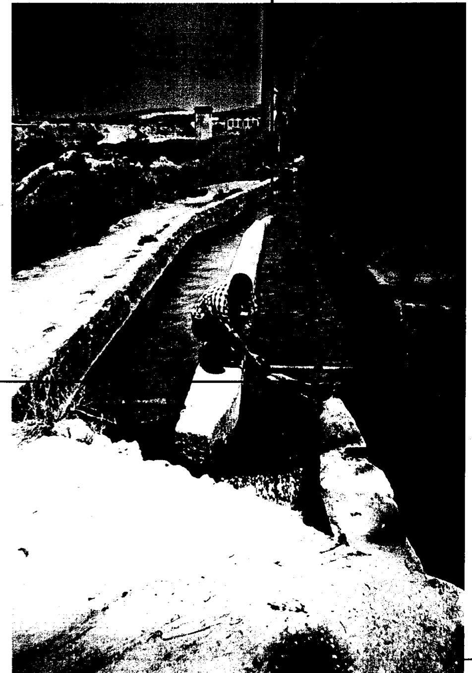
Anoi has a second mobile partidor. This allows Anoi irrigators to sell a part of their water to irrigators placed downstream in the hydraulic system
