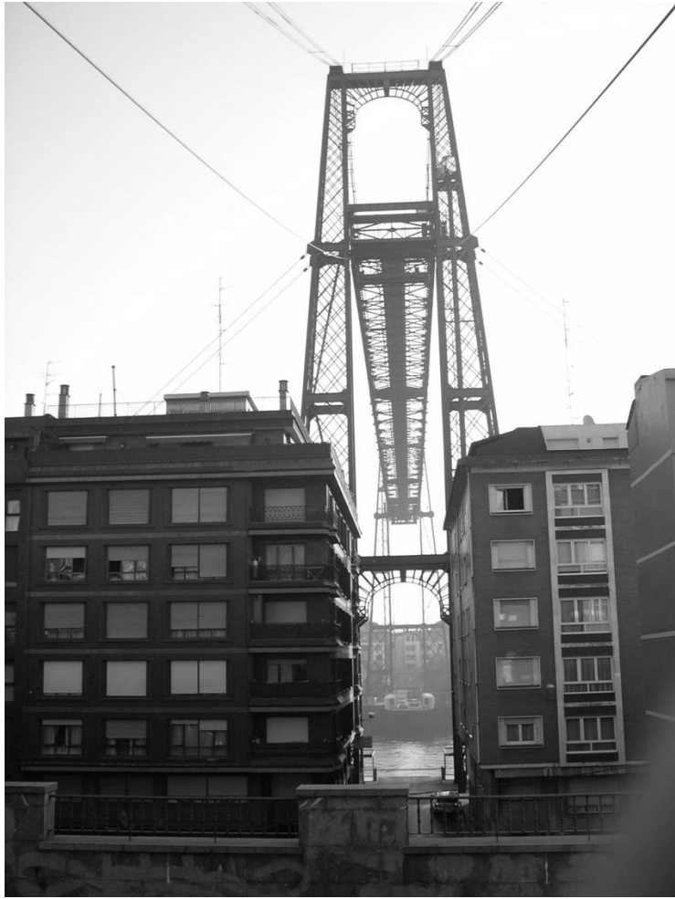
Bridge from the street
