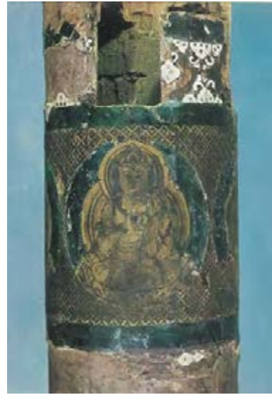
photo 2-14 Image of Buddha on the pillar (upper section) (before repair work)
