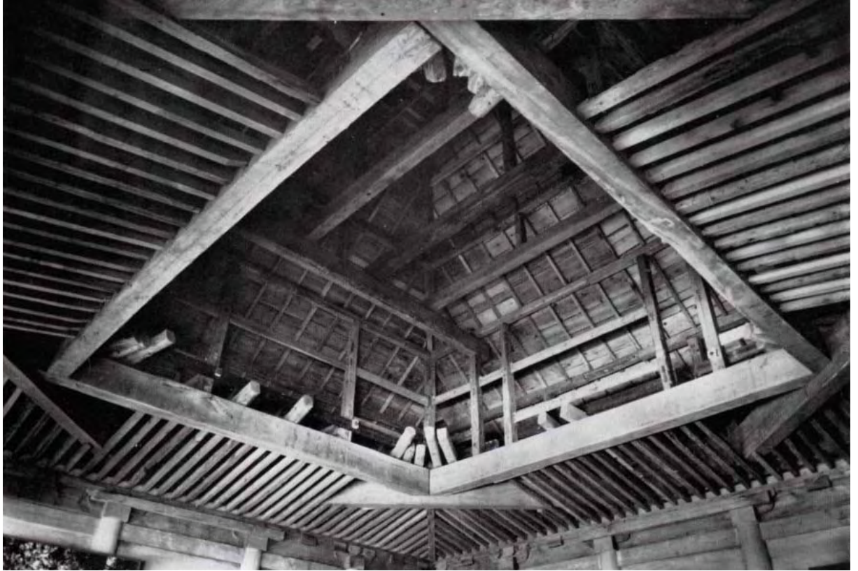
photo A4-17 Roof structure of Konjikidô Ôidô (inside) ©Chûson-ji
