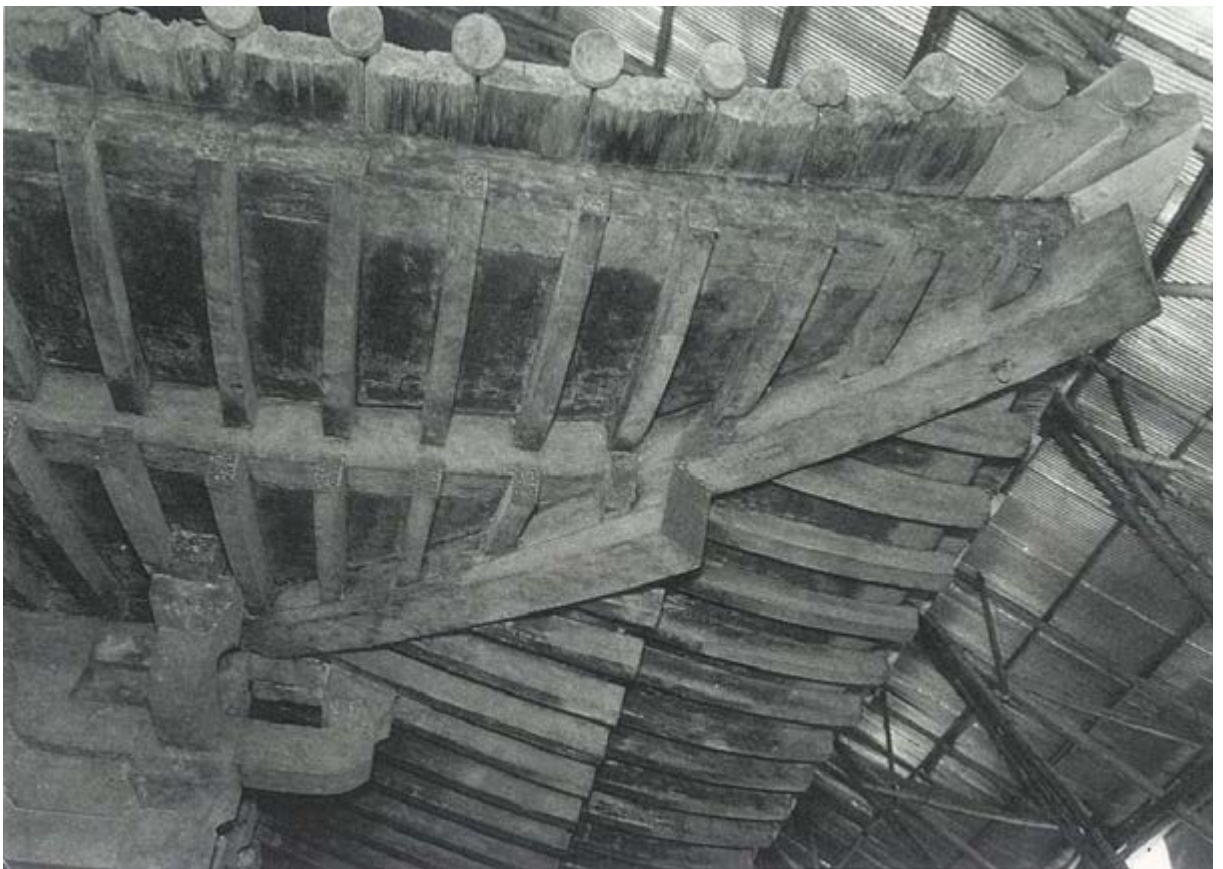
photo A4-4 Eaves of Konjikidô before dismantling ©Chûson-ji
