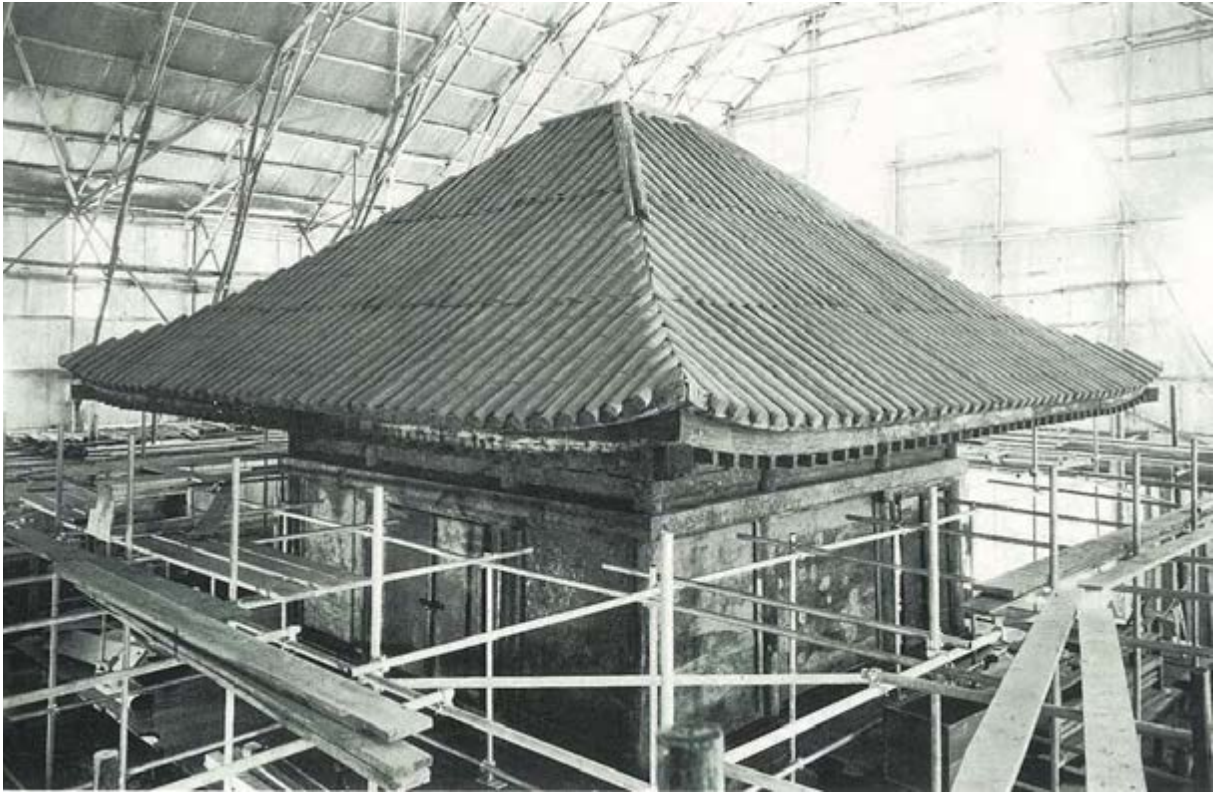
photo A4-3 Roof of Konjikidô before dismantling ©Chûson-ji
