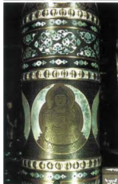
photo 2-16 Image of Buddha on the pillar (lower section) (after repair work)
