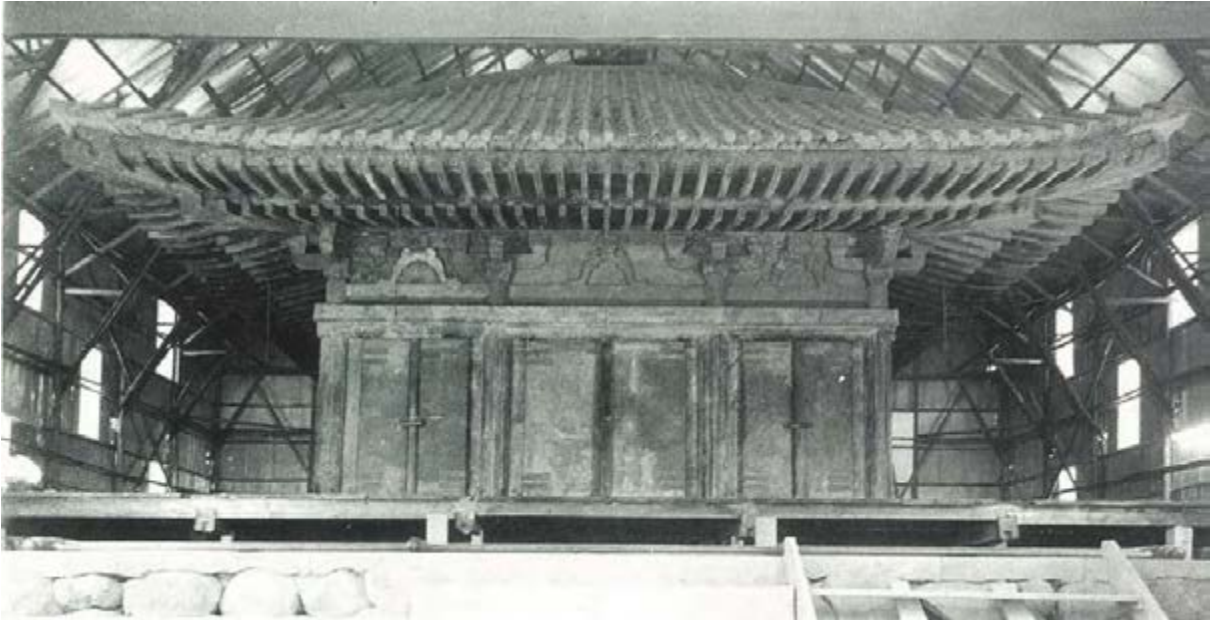
photo A4-1 Konjikidô before dismantling (front) ©Chûson-ji
