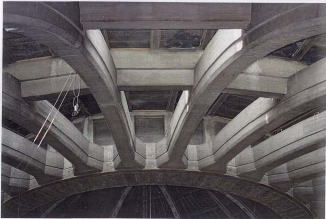
51. Centennial Hall, interior, ribs of the dome, contemporary photograph.
