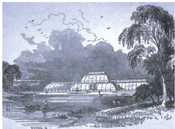
7.3.5 Exterior of the Palm House [3012], 19th century
