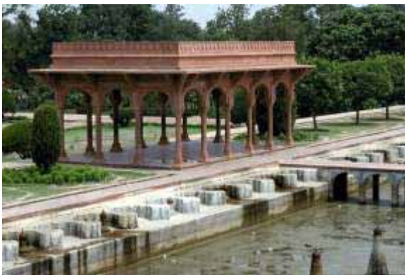
The reconstructed red sandstone Pavillion
