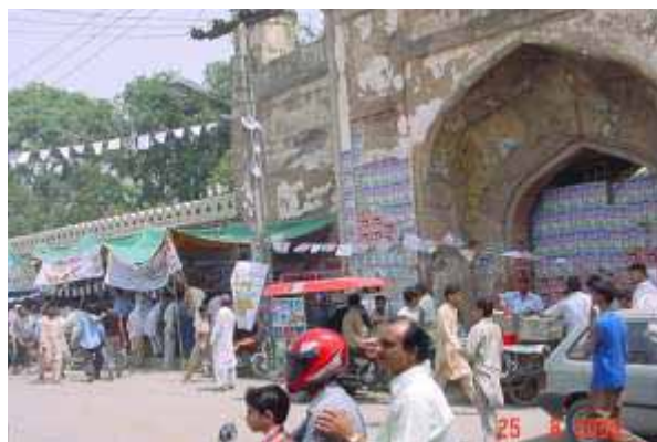
Deteriorating frescoes of the Shahi Hamam
