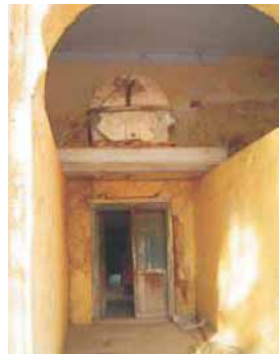
Unacceptable toilet facilities inside the Shahi Hammam
