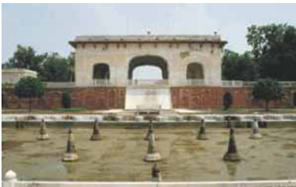
The Aiwan and Main Tank
