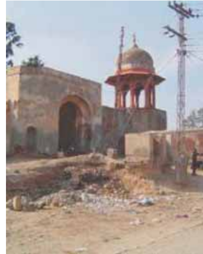
Garbage and utilities damaging the Exterior of the World Heritage site
