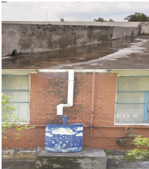
Rain water catchment: harvested water being stored in multiple use
