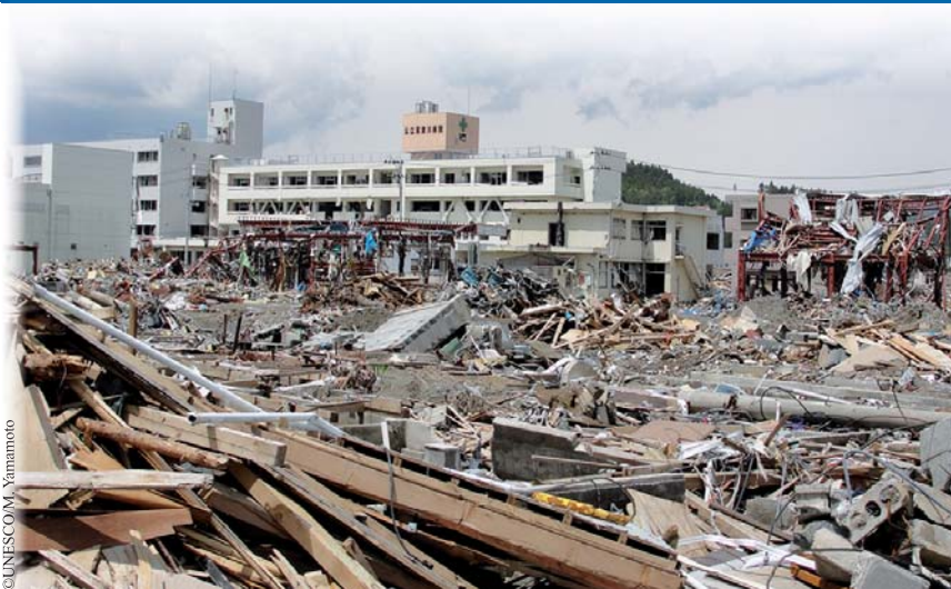
View of the hospital in Minami-Sanriku in May, one of the rare buildings left standing. The tsunami waves only spared the top floor. Of the 107 patients, 72 died. Most of the victims were elderly and needed help to evacuate. To make matters worse, the elevator was out of order following a power cut caused by the earthquake. The earthquake caused the ground in the region to subside by about 1 m.
