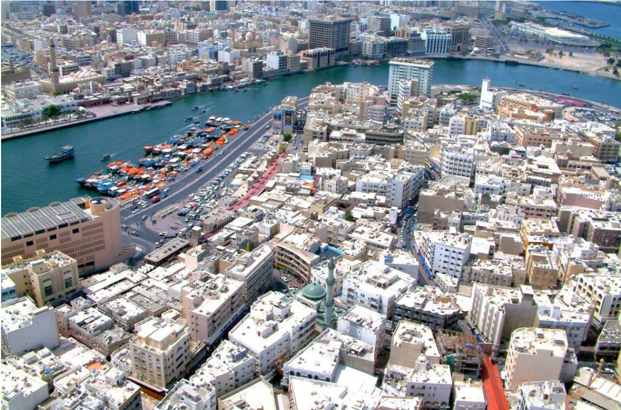
General view of the nominated property
