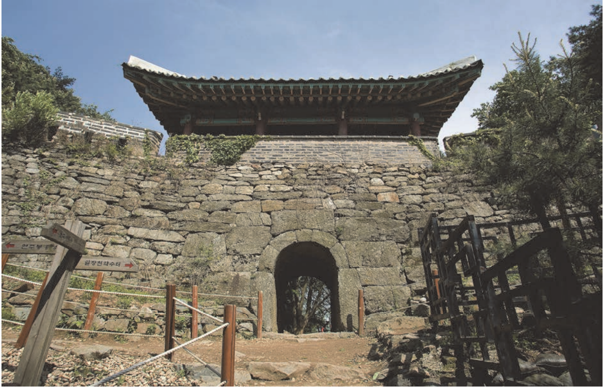
The eastern gate
