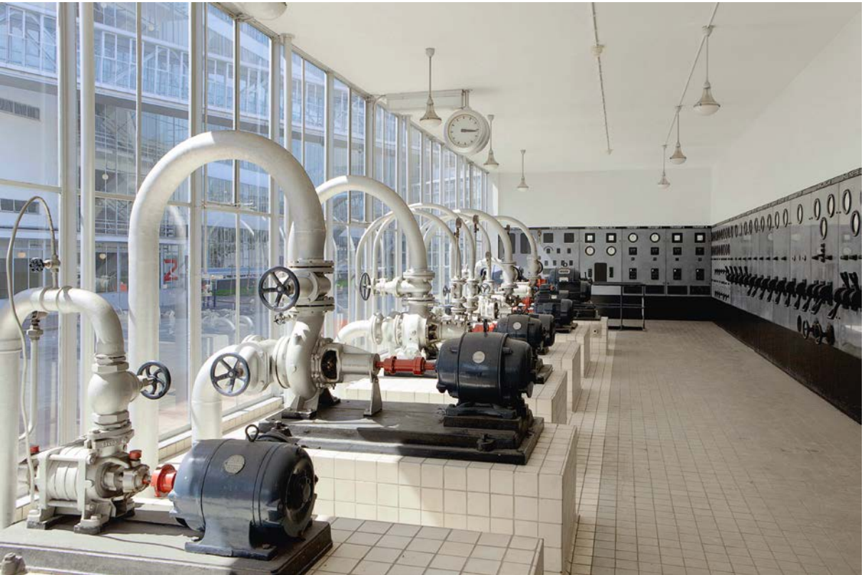
The boiler house
