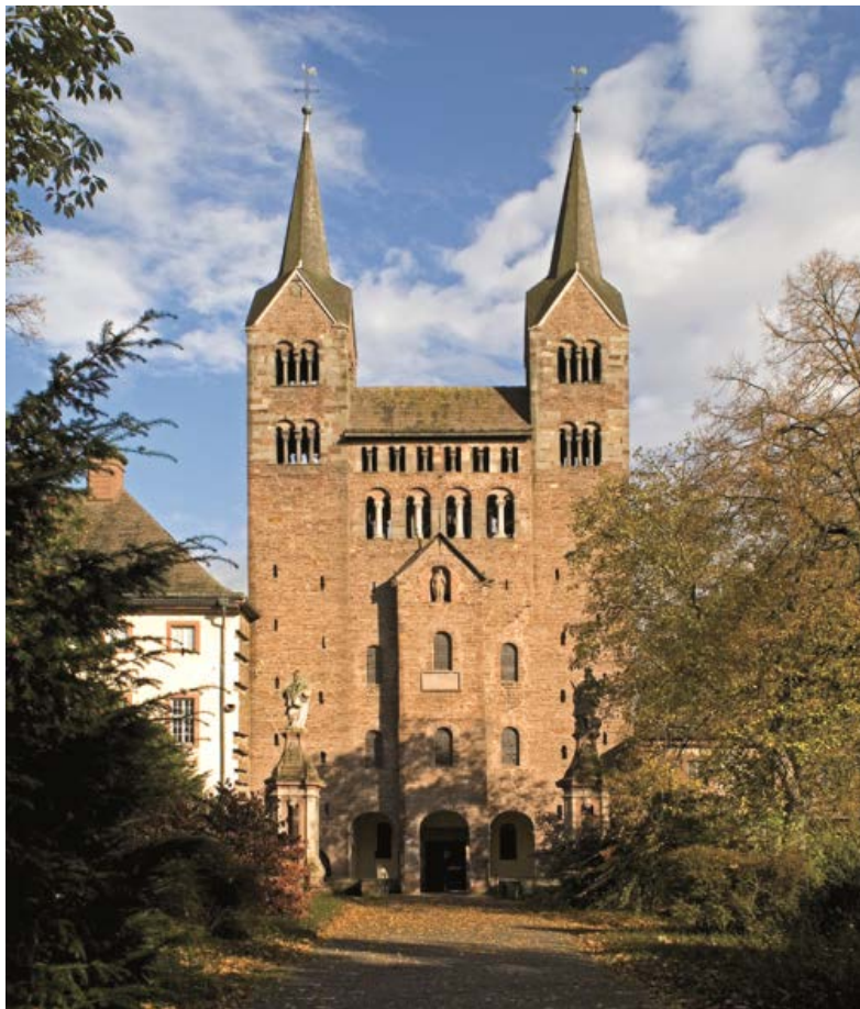
View of the Westwork of Corvey
