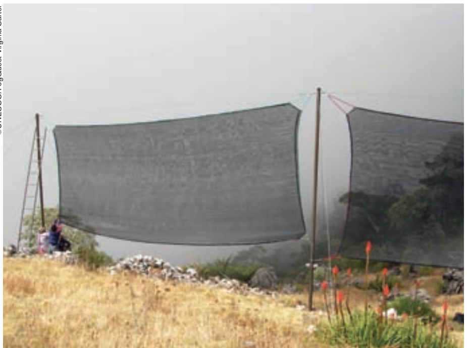
Fog collectors being constructed in La Ventana, Guatemala
