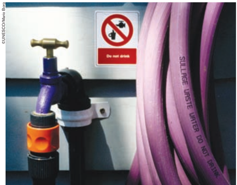
Hose for sullage waste water, Melbourne, Victoria, Australia.
