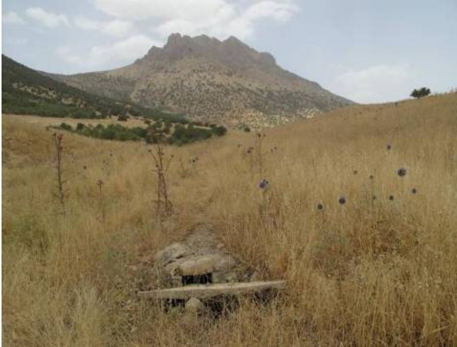
Figure 2. Cut-and-cover section of canal at the outflow of a karez at Basak. (Photo by Dale Lightfoot)
