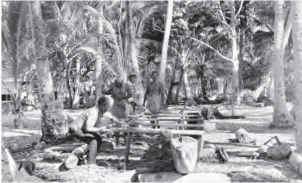
Attaching an outrigger to a canoe
