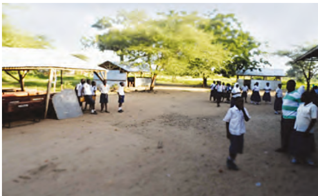
Temporary classrooms at Magole Primary School at Morogoro. © UNESCO National Commission of the United Republic of Tanzania
