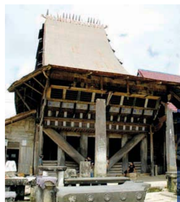
Traditional architecture with higher earthquake resistance © Dandi Prasetya
