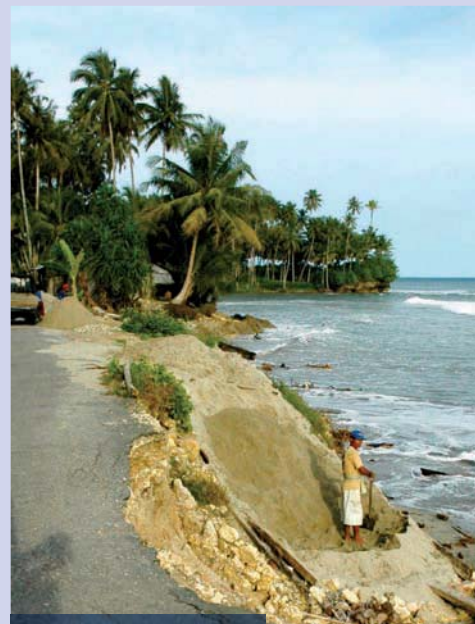
Coastal erosion endangering coastal infrastructure in Nias © Jan H. Steffen
