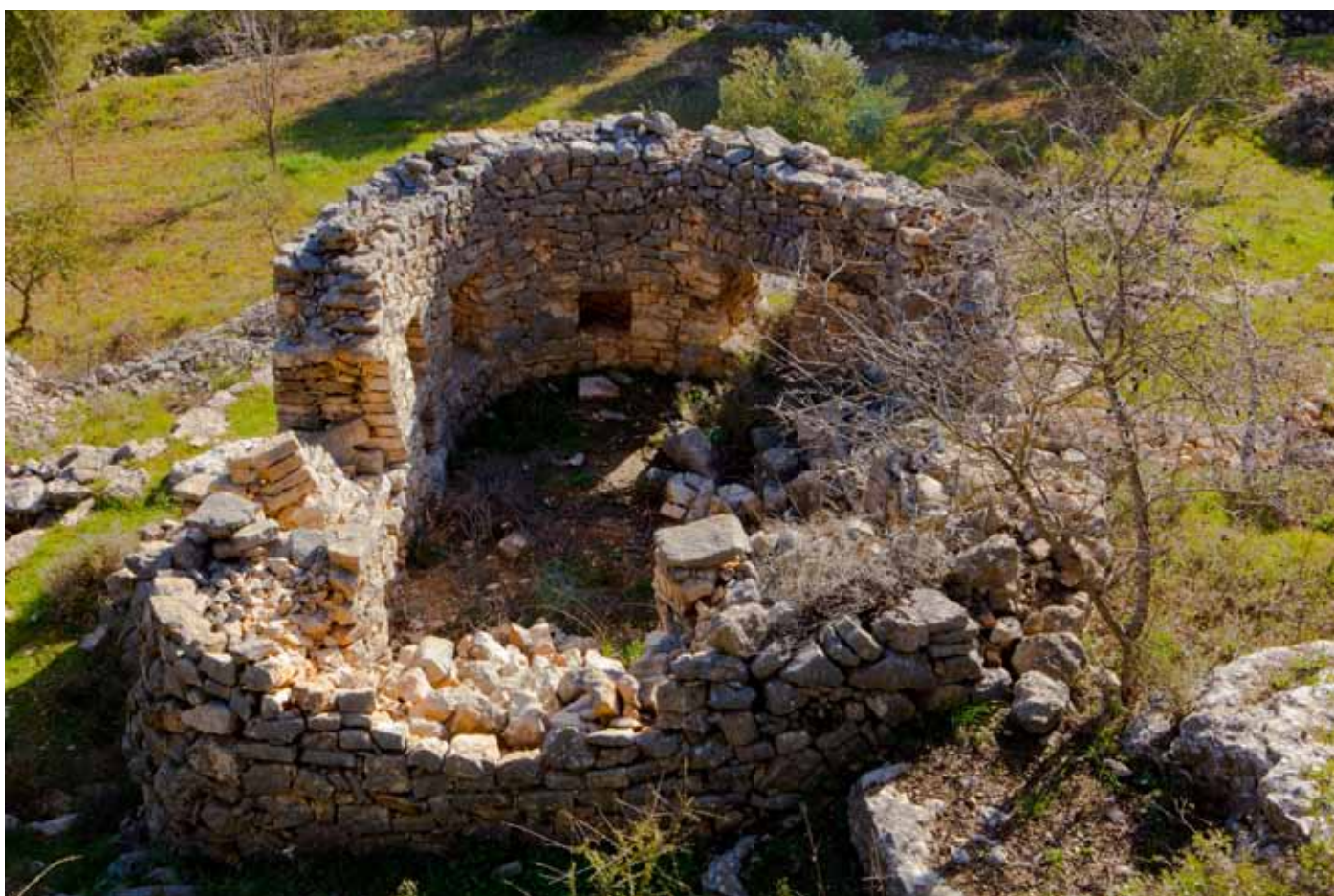
Fig 4.3 A watchtower with a collapsed roof near Wadi Al-Makhrour
