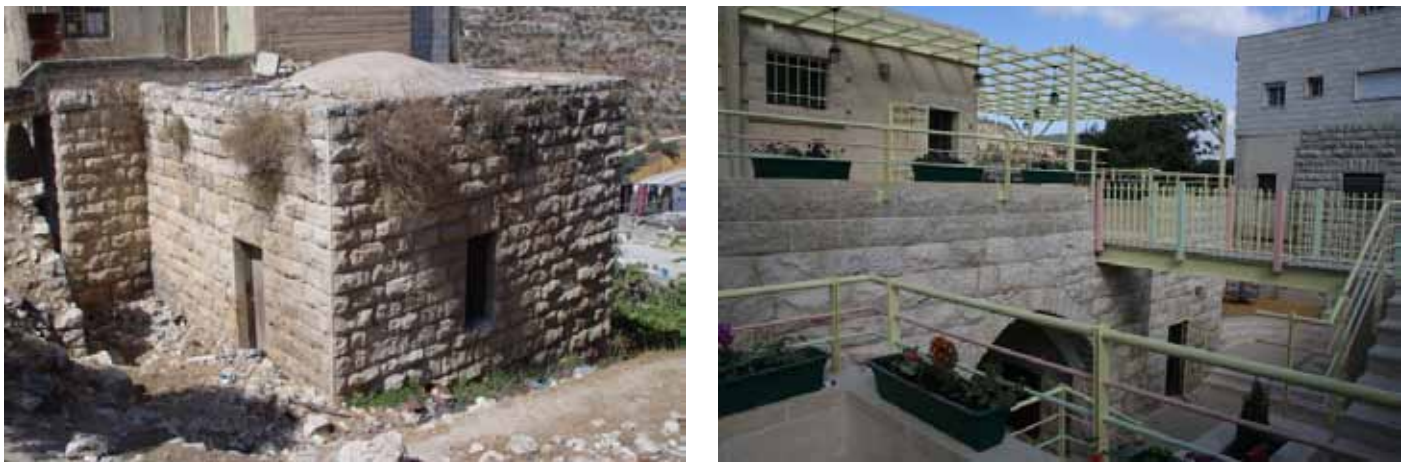
Fig. 2.27 Dar Al-Bader before and after renovation
