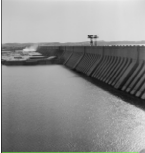
ASWAN DAM ON NILE RIVER
