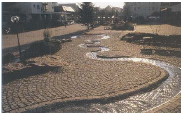
Figure 1 Open channel used for rainwater transfer in Germany
