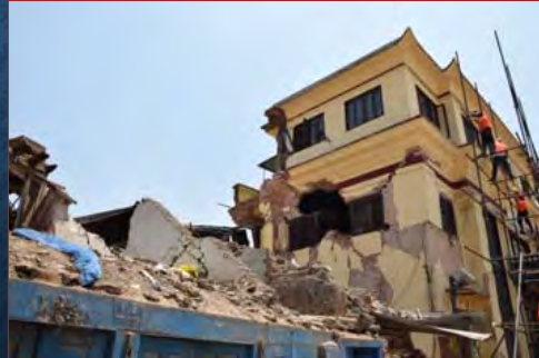
After Earthquake ruined surrounding area
