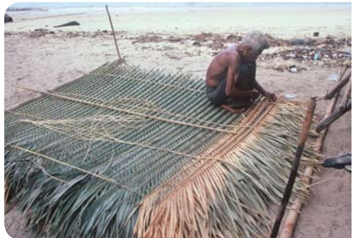
Photo 10: Making thatched roof from nipa palm
