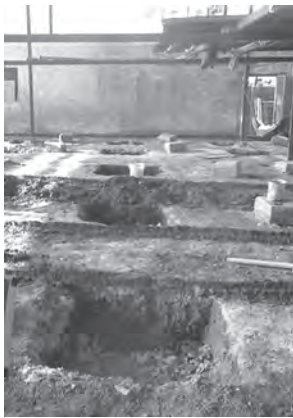
Figure 6-19b: Repair work to fix uneven subsidence of foundation / Sửa chữa lún móng
