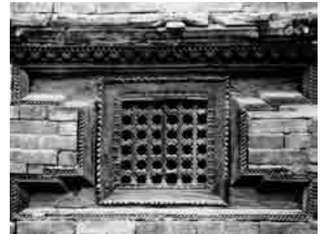
Fig. 72 Glazed shutter in lattice window.
