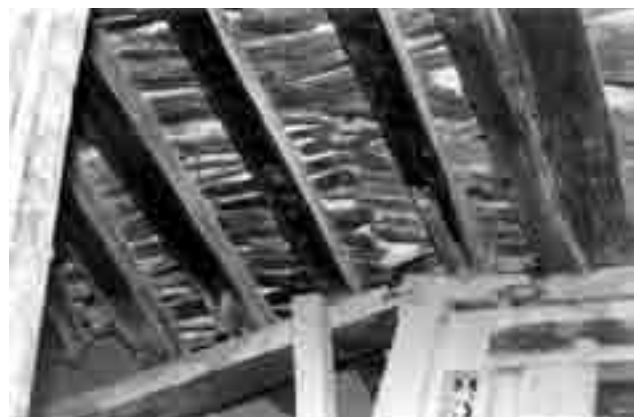
Fig. 97. Laths above the rafters.
