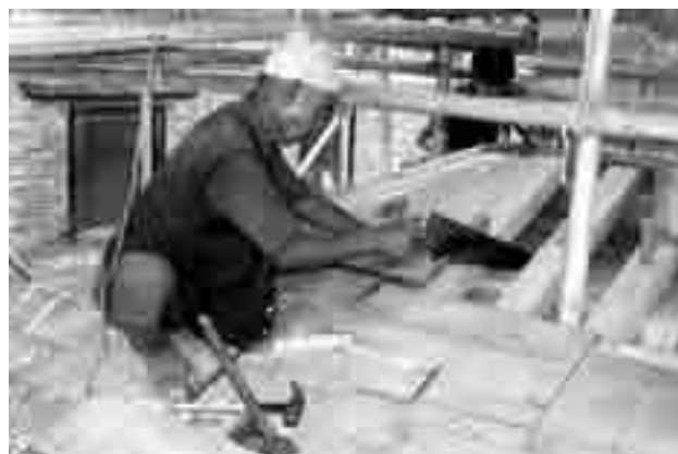
Fig. 98. Planking above the rafters.
