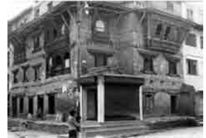
Fig. 33. Juxtaposition of modern and old structure.
