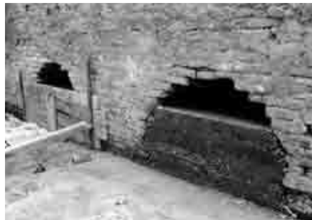
Fig. 88. Inserting damp proof course.
