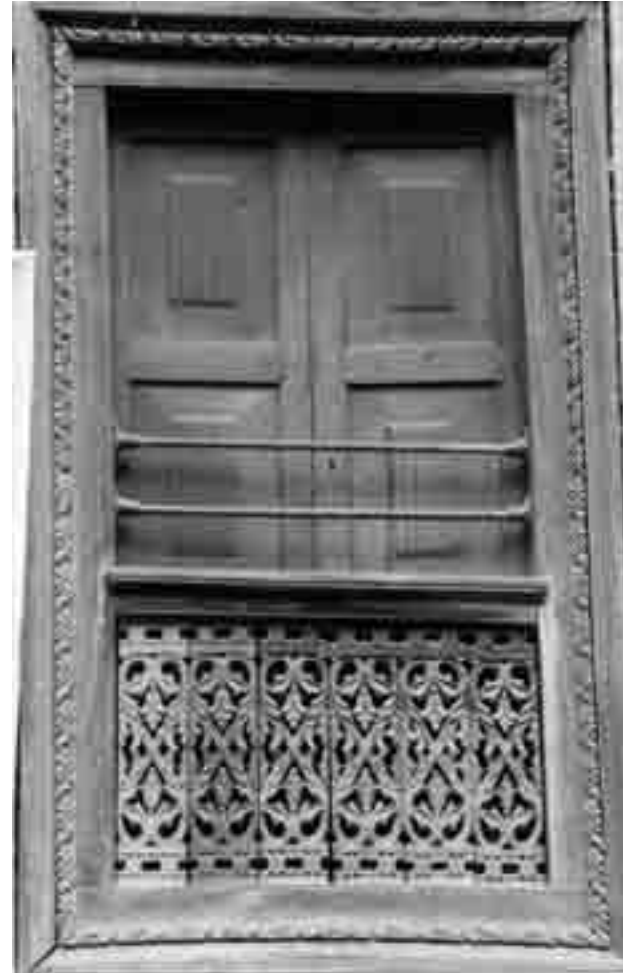
Fig. 70. Repair of carved elements.
