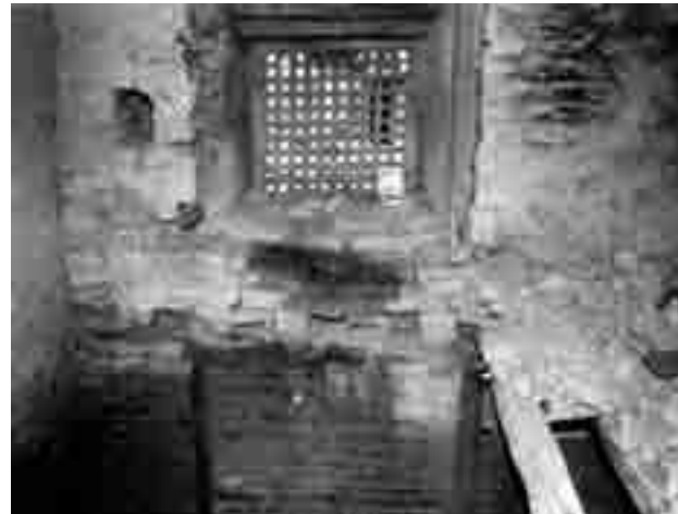
Fig. 49. Damage from ground damp.
