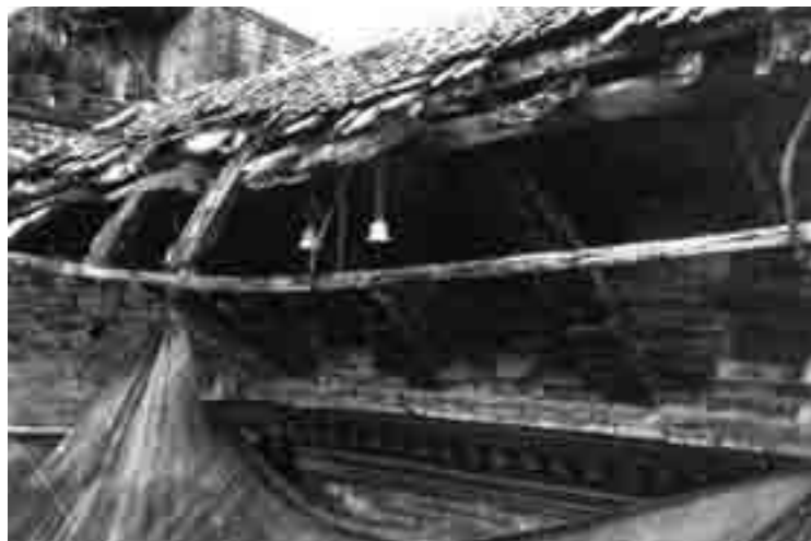
Fig. 51. Decay of eaves board.
