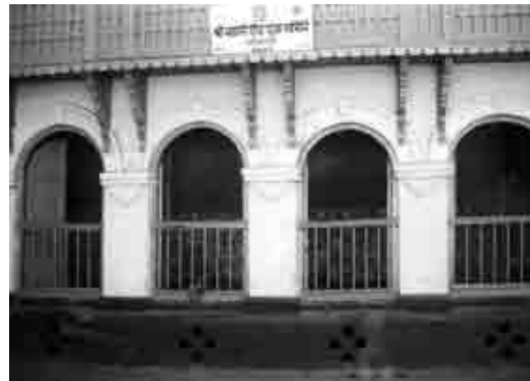
Fig. 84. Air holes for air circulation.
