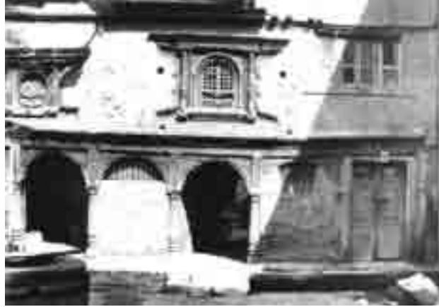
Fig. 62. Settlement of beam.
