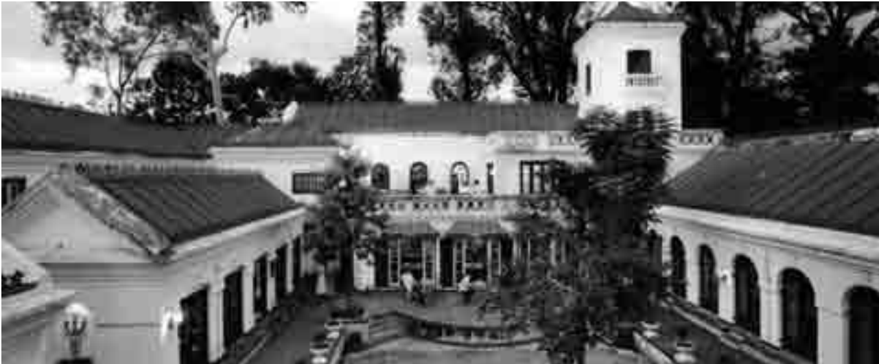
Fig. 25. Adaptive re-use for shopping complex.
