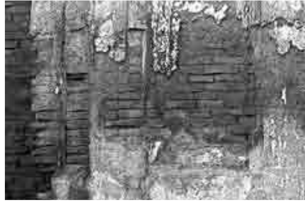
Fig. 100. Damage to plaster by ground damp.
