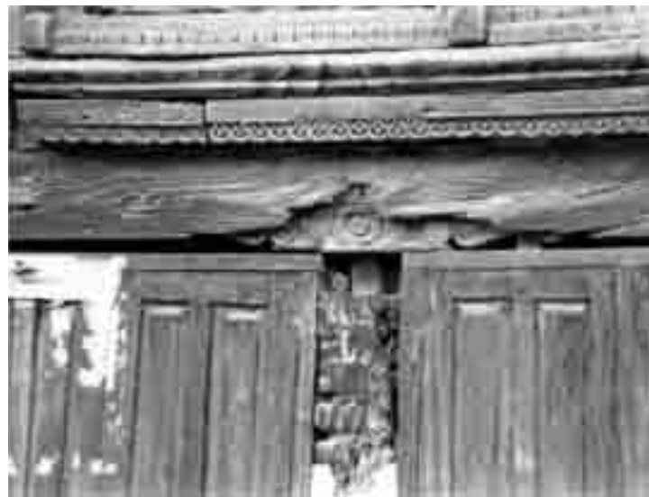
Fig. 44. Deterioration of timber elements from insects.
