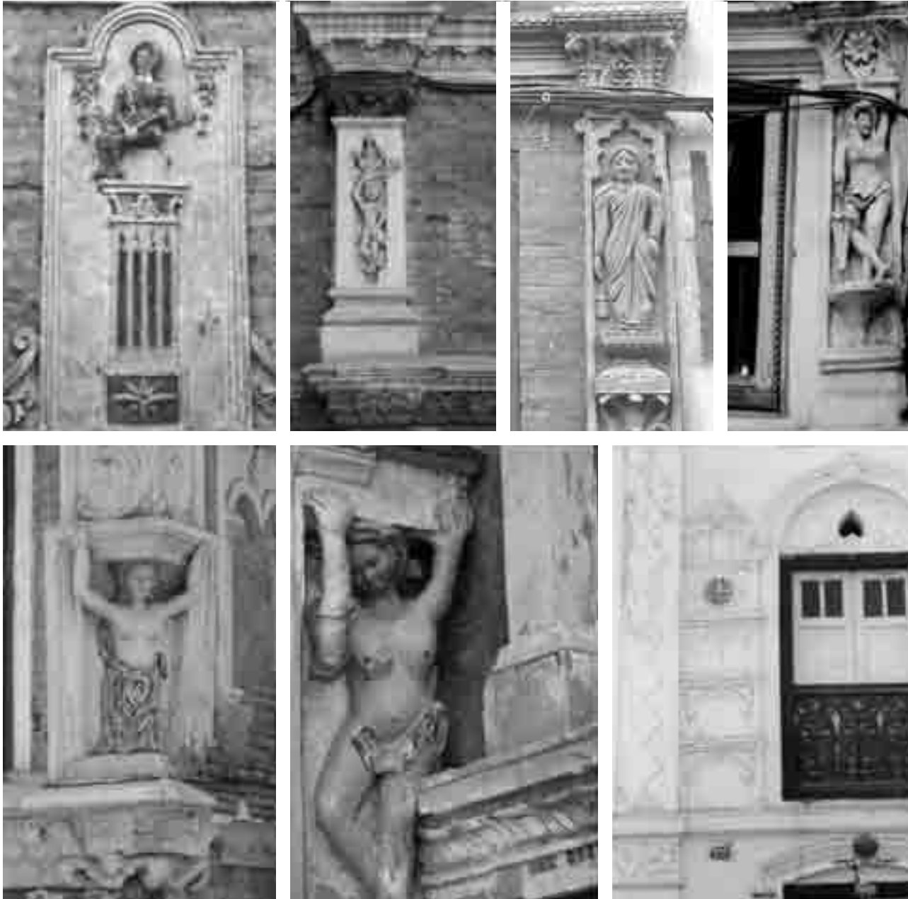
Fig. 102. Examples of ornamental plasterworks.
