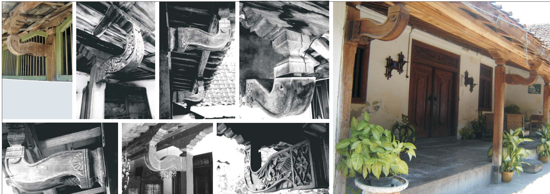
Fig. 38: Bahu dhanyang variations in Kotagede Gbr. 38: Ragam bahu dhanyang di Kotagede
