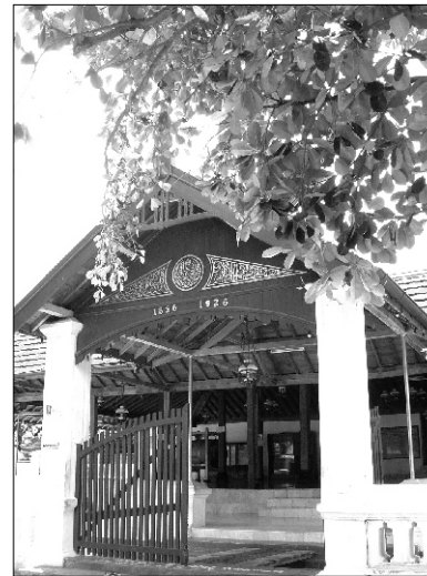
Fig. 22: Main entrance of Kotagede Grand Mosque Gbr. 22: Pintu utama Masjid Agung Kotagede
