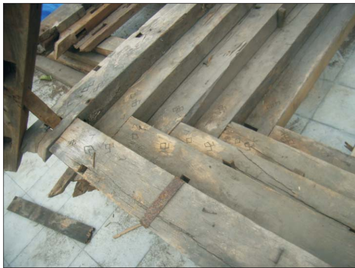
D6 Fig. 78: Detail D6, joint between blander pamidhangan pamanjang and pamidhangan panyelak Gbr. 78: Detil D6, sambungan antara blander pamidhangan pamanjang dan pamidhangan panyelak
