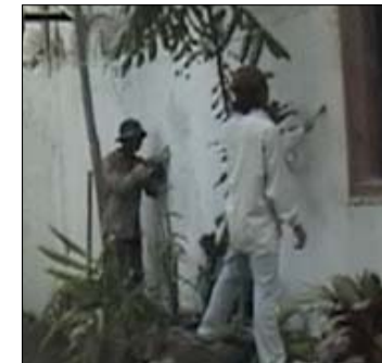
Fig. 111: Cleaning before painting Gbr. 111: Pembersihan sebelum pengecatan
