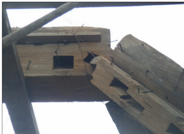
D8 Fig. 80: Detail D8, joint between molo and dudur brunjung Gbr. 80: Detil D8, hubungan antara molo dan dudur brunjung
