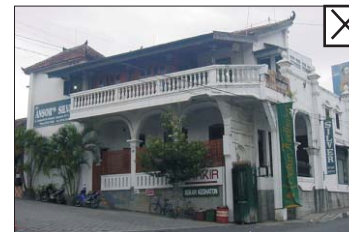
Fig. 147: Building height that exceeds 8 m is inappropriate Gbr. 147: Ketinggian bangunan yang melebihi 8 m
