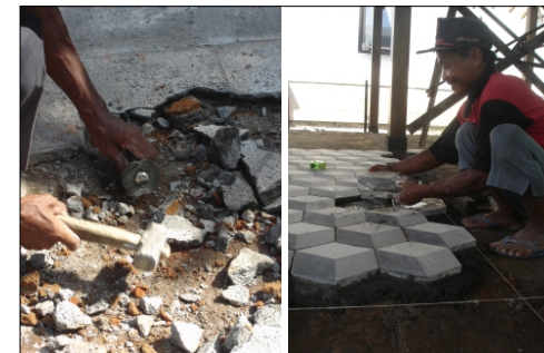
Fig. 175: Removal of old floor and installation of new floor
