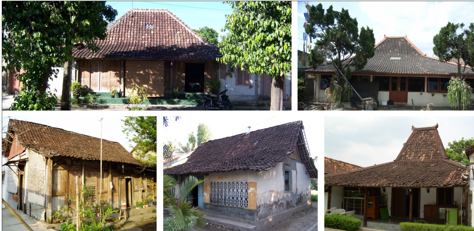
Fig. 51: Various kotangan walls Gbr. 51: Ragam dinding kotangan
