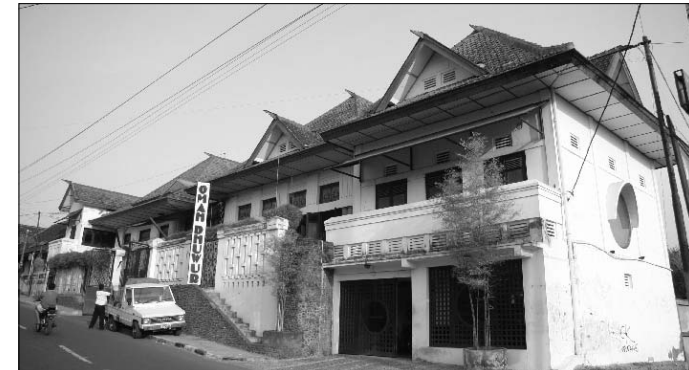
Fig. 25: A shop house belonging to a wealthy merchant in Mondorakan Street Gbr. 25: Toko milik pedagang besar di Jalan Mondorakan
