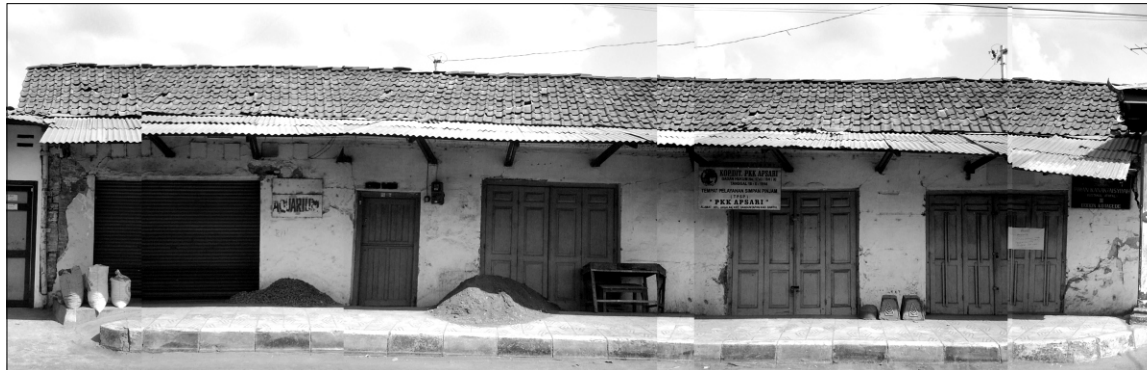
Fig. 24: A shop house belonging to an ordinary merchant in Mondorakan Street Gbr. 24: Tipe rumah toko pedagang dari kalangan biasa di Jalan Mondorakan
