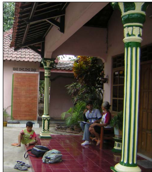
Fig.104: Shiny ceramic floor is not recommended Gbr. 104: Lantai keramik mengkilap tidak direkomendasikan
