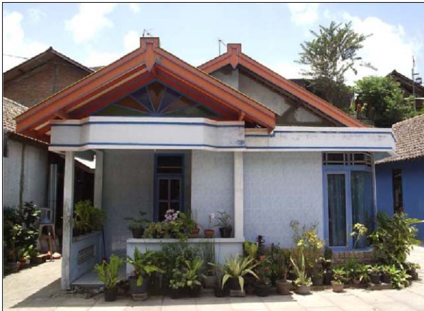
Fig. 106: Flat roofs (concrete) are not recommended Gbr. 106: Atap datar (dak beton) tidak direkomendasikan
