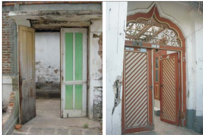
Fig. 113: Butulan door of rukunan street Gbr. 113: Pintu butulan di jalan rukunan
