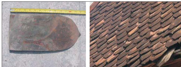
Fig. 61: Clay shingle roof tiles Gbr. 61: Genteng sirap tanah liat
