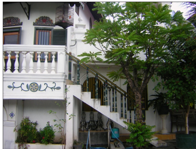
Fig. 136: Ornamented concrete staircase of a Kalang house
