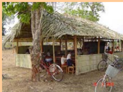
A temporary school in Preah Vihear
