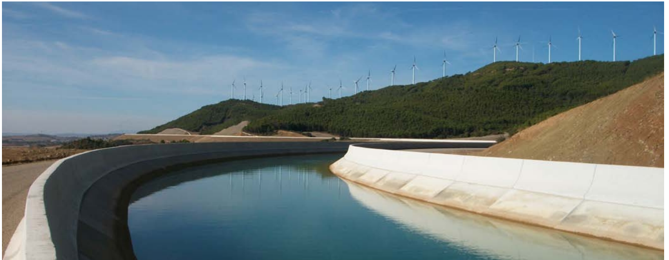
Fig. 2. Navarre irrigation channel.
