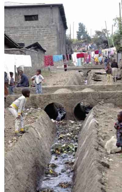
Open sewers in slum area of Addis Ababa, Ethiopia
