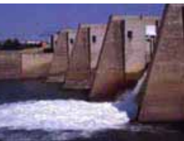
Pierre Bénite dam, France
