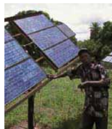
This solar voltaic panel's energy is used to pump water, Kabekel village, Gambia
