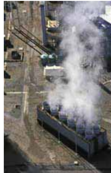
Aerial close-up of Tucson Electric Power's cooling towers, Arizona, United States
