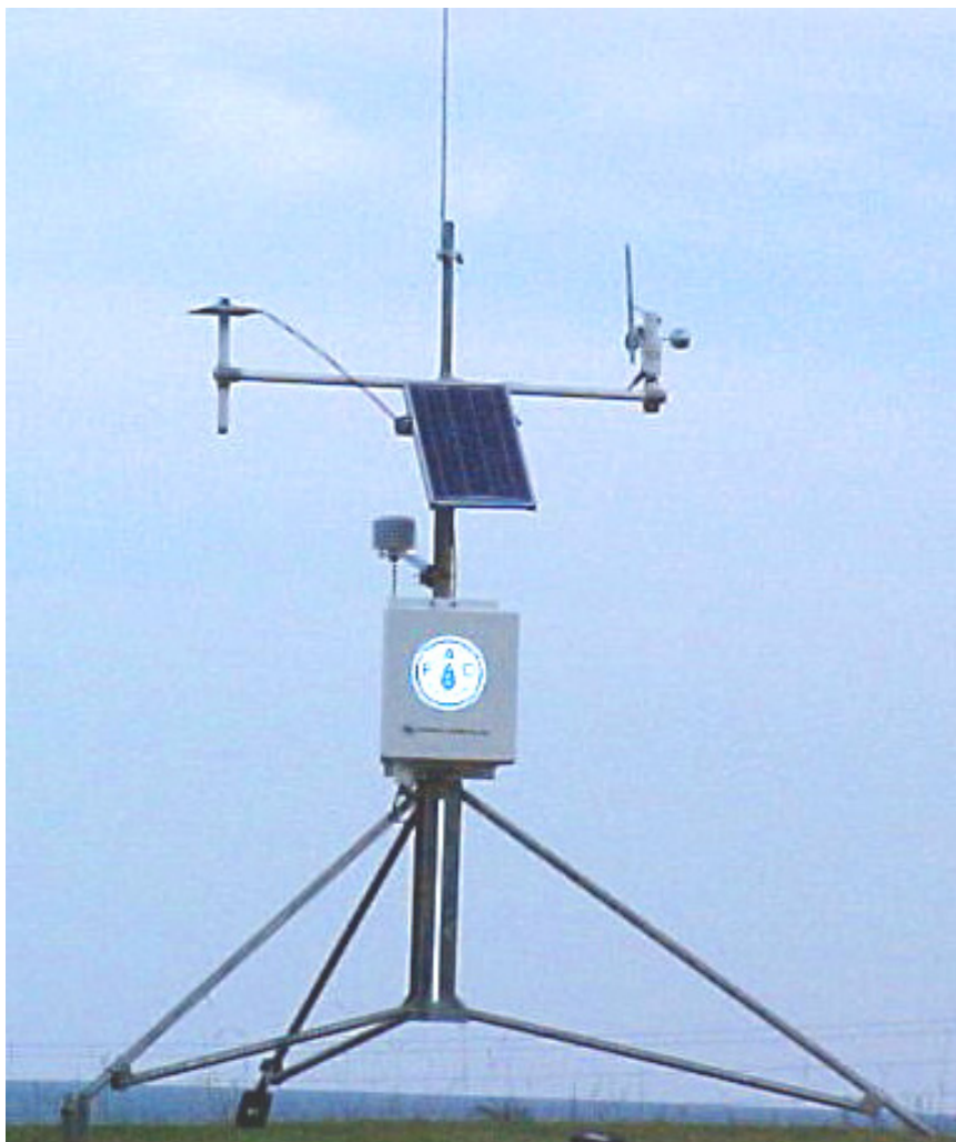
Figure 3.10 – Typical Automatic Weather Station
