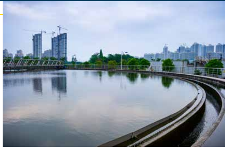
Modern urban wastewater treatment plant Photo: © hxdyl/Shutterstock.com
