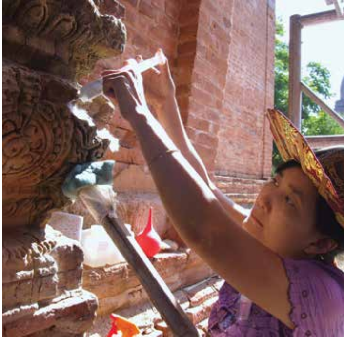
© UNESCO/R. Lujan Consolidating the stucco at the Hsin-bbyiu-shin monastic complex. Myanmar Consolidation du stuc au sein du complexe monastique Hsin-bbyiu-shin. Myanmar Consolidação do estuque no complexo monástico Hsin-bbyiu-shin. Myanmar
