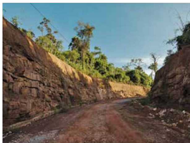
A road newly built through a jungle in Koh Kong province.
