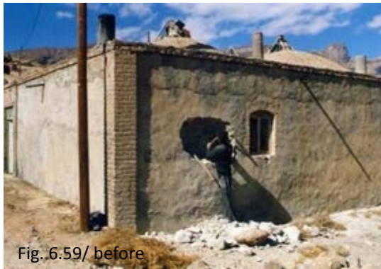
Fig. 6.59/62 New bath before and after conservation activities within 1381/2002 and 1383/2004
