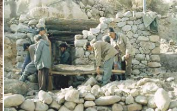
Fig. 2. 105 Rezmalek Water-mill being repaired
