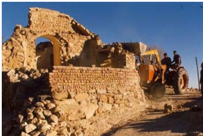
Fig.4.9 Destructing inappropriate buildings, considering the integrity of troglodyte Maymand
