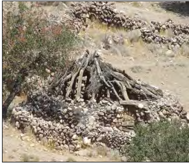
Figs. 2. 91 Gombeh's roof structure with convergent beams
