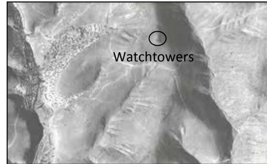
Fig.2. 113 Watchtower in Maymand 's aerial photograph
