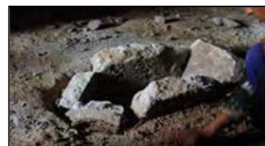
Fig.2.181 Securing stones with mud mortar
