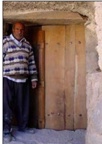
Fig.2.192 A double-leaf door (made by master carpenter Habibollāh Ebrāhīmī)
