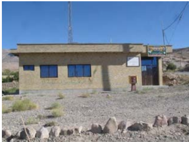
Fig.4.82 The construction of post office which is inappropriate with troglodyte fabric of Maymand
