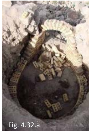
Fig.4.32.a/f Process of establishing half cooking calk kiln
