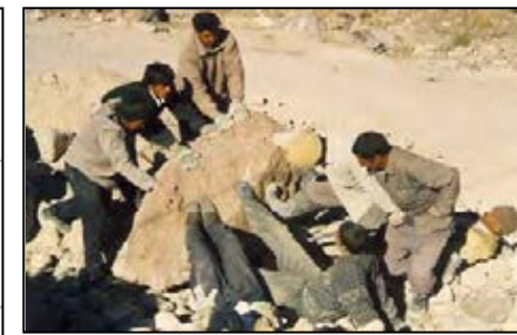
Fig.2. 215 Holding on to the stone in an unstable position using hands and feet
