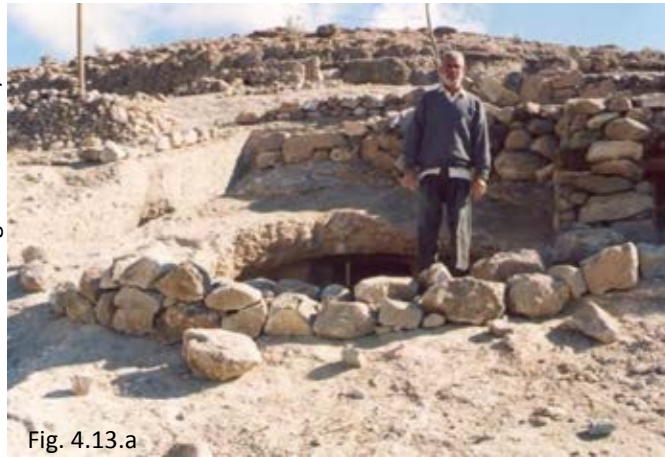
Fig.4.13.a,b Different process of restoration of damaged roof 1380/2001
