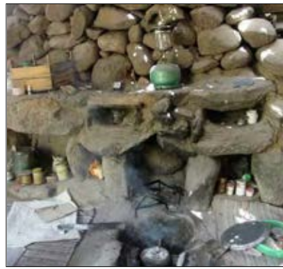
Fig. 2. 93 Part of the internal space of a Gombeh , Didān and stone niches
