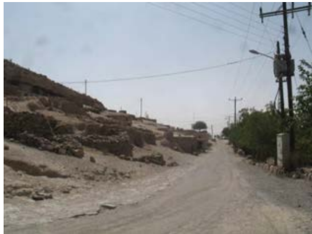
Fig.4.93 Inappropriate pole with the visual integrity of troglodyte Maymand
