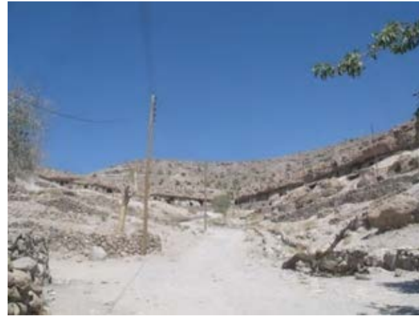
Fig.4.94 Inappropriate pole with the visual integrity of troglodyte Maymand
