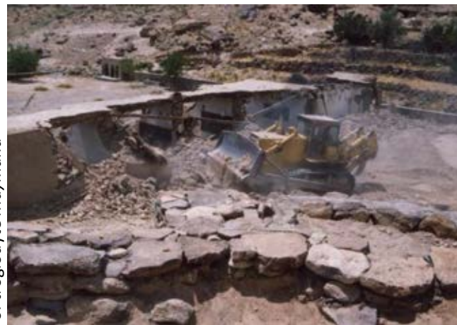
Fig.4.10 Destructing inappropriate buildings, considering the integrity of troglodyte Maymand
