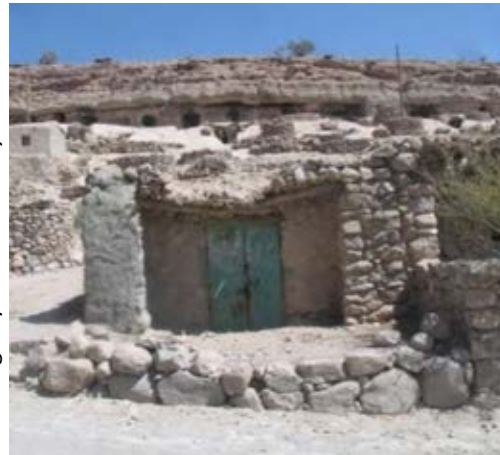
Fig.4.86: An inappropriate construction with troglodyte fabric of Maymand
