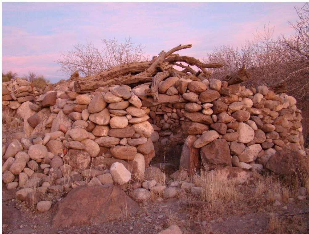
R2.Fig. 27: A summer hut or Gombéh constructed of rubbles in walls and timbers in roof
