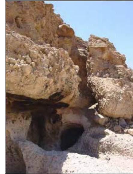
Fig. 2,384 Destruction of raised layers of Tāq as the result of lightning.
