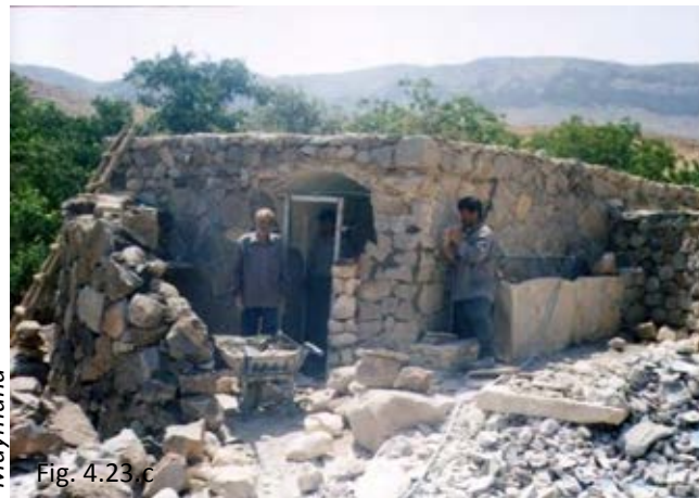
Fig.4.23.a/d Improving public toilets near the mosque in troglodyte Maymand
