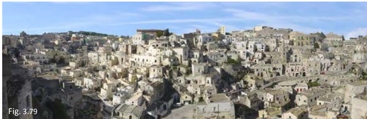
Fig. 3.79,80 General view of Matera
