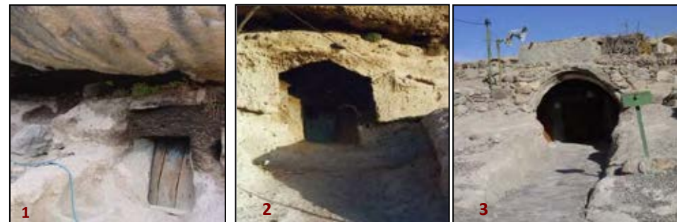
Figs. 2.145 Different Eyvān types in terms of form: 1- naturally formed Eyvāns in Pātāq 2- Carved Eyvān in Kamar 3- Eyvān with a break-made roof
