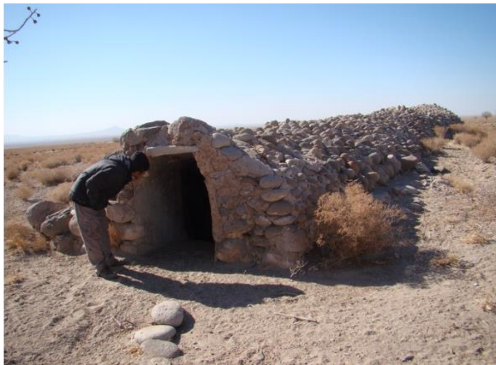
R2.Fig. 28: A reservoir with barrel roof in eastern bank of Maymand River
