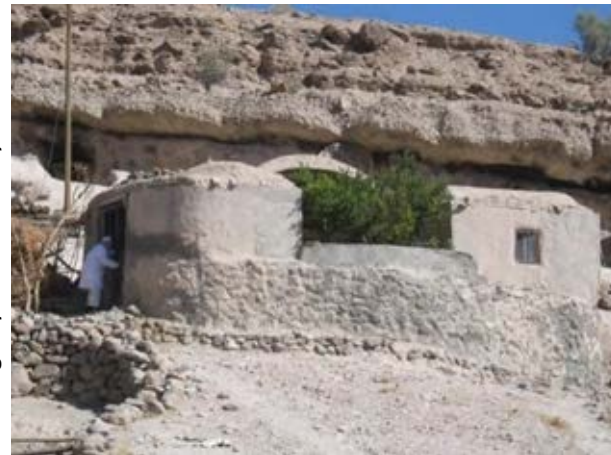
Fig.4.89: An unsuitable structure with troglodyte fabric of Maymand
