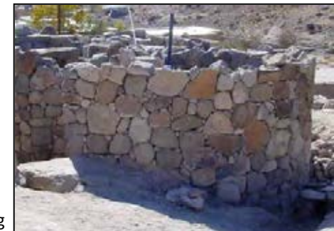
Fig. 2, 224 Using display stones in wall-making
