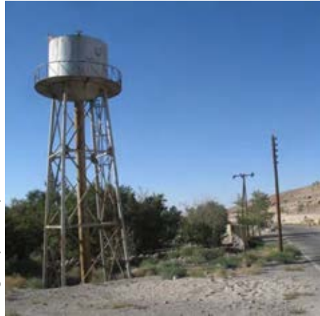
Fig.4.90 The water supply place which is considering the integrity of troglodyte Maymand
