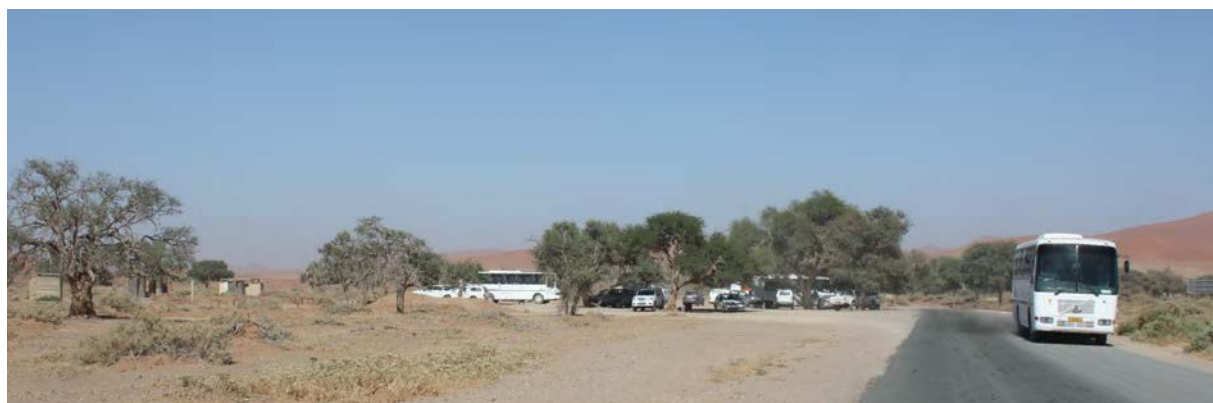
Figure 4.b.3: Heavy tourism traffic to Sossus Vlei 2x4 parking lot warranted a 60 km tarred road to reduce dust and ease road maintenance (Gobabeb Centre)
