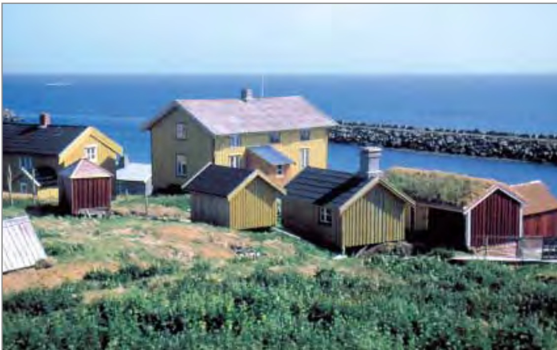
50. The houses on Skjærvær have recently been refurbished. June 2002.
