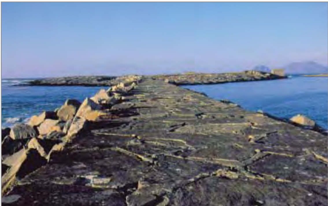
60. Breakwater on Bremsteinvær. June 2002.
