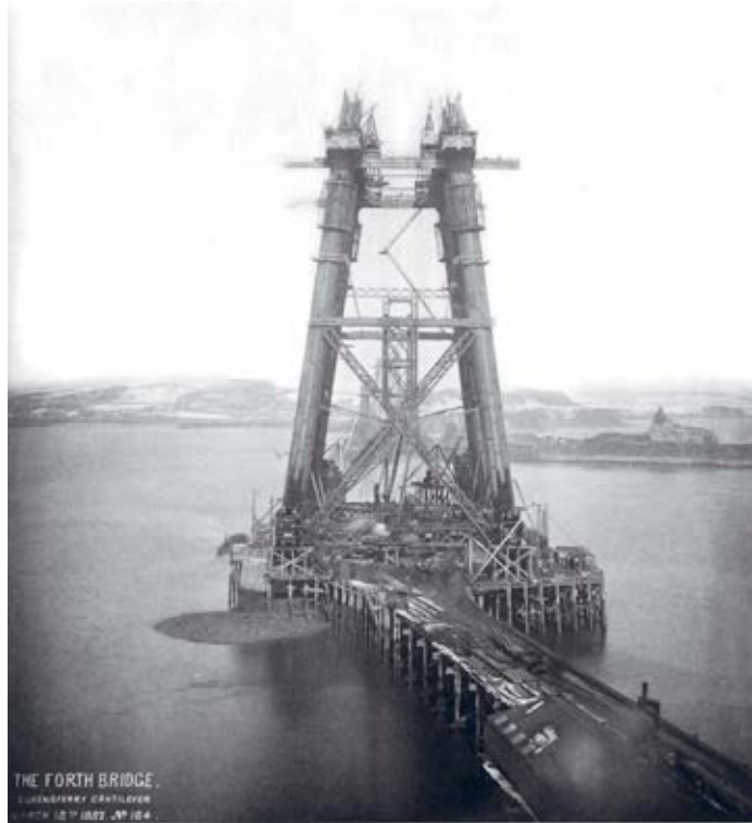
Photograph showing progress of the Queensferry main tower
