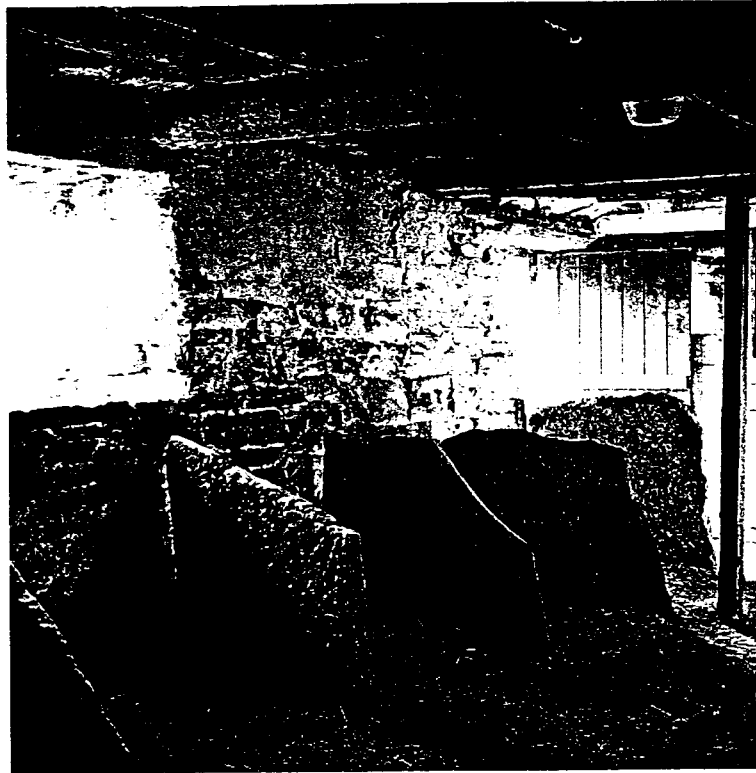
Photo 51 Limestone, easily extracted and near at hand, was used for both buildings and fittings – here as stall partitions. Anders Johansson.
