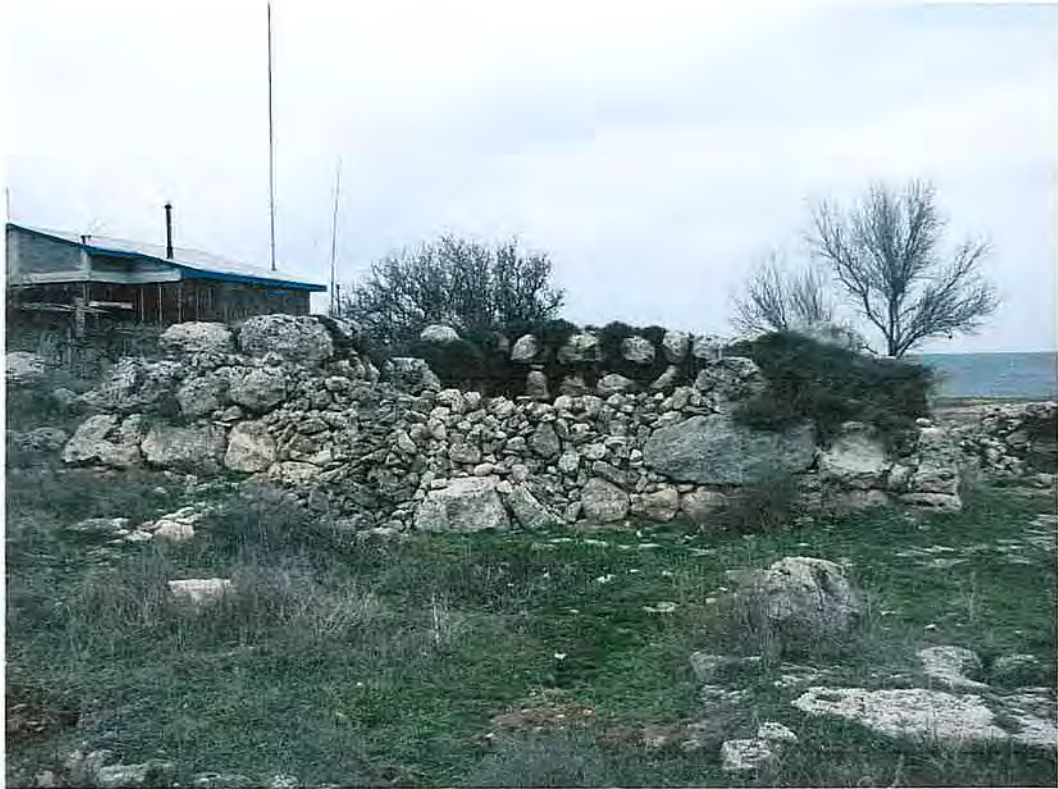
Fig. 11. Ancient antiseismic wall strengthening constructions on an ancient farmstead in the Chersonese chora
