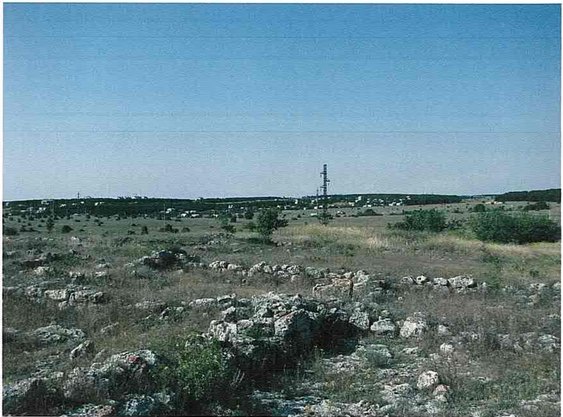
Fig. 18. Dissonant power transmission tower on the protected site in the Yukharina Gully
