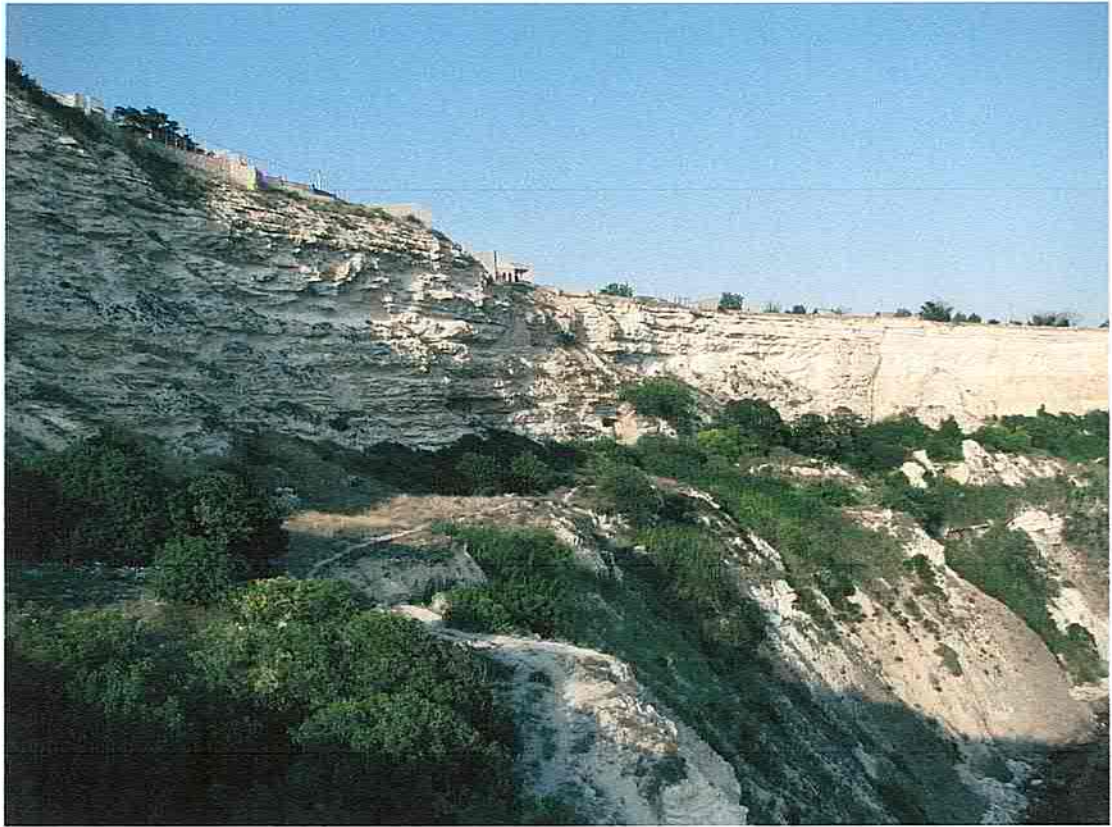
Fig. 13. Terrace and cave constructions on Cape Vinogradny damaged by a landslide
