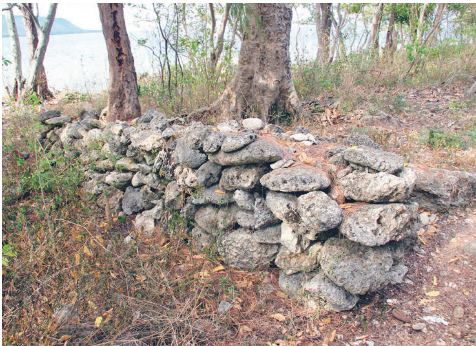
Figure 3.2 Stone wall, Lelepa Island
