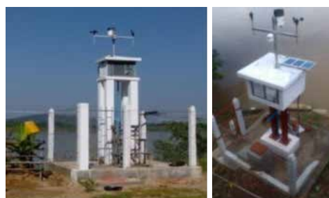
Figure 6.8.1. Hydrometry Monitoring Systems. Photo ©IHP Myanmar
