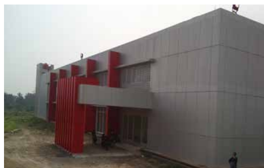
Figure 7.1.6. APCE Building. Photo ©APCE
